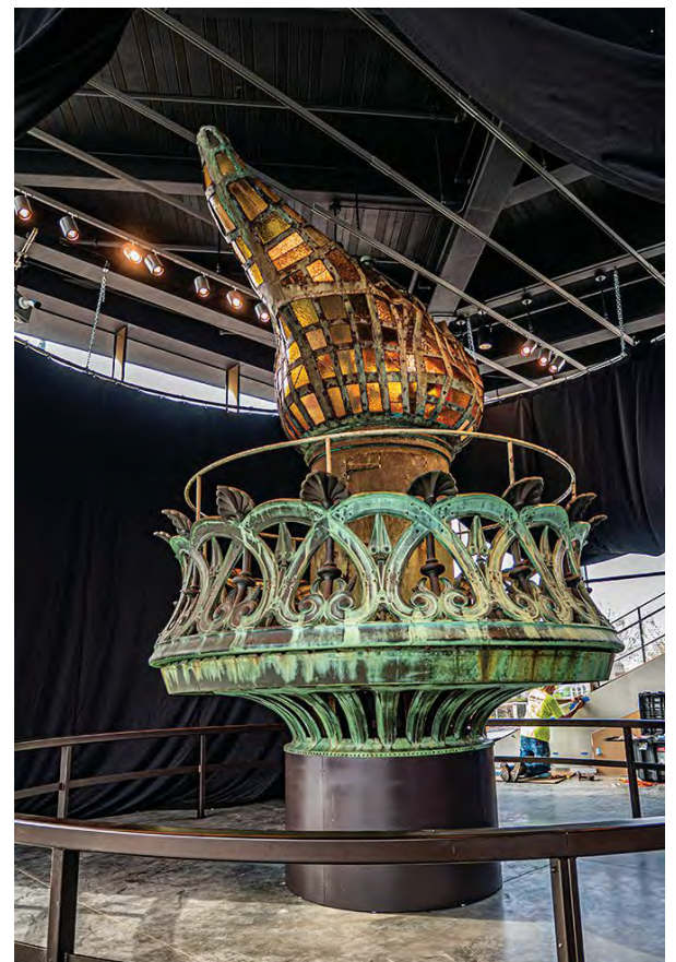
The flame dates to the 1916 redesign with hundreds of amber glass pieces in a repousse copper shell.
