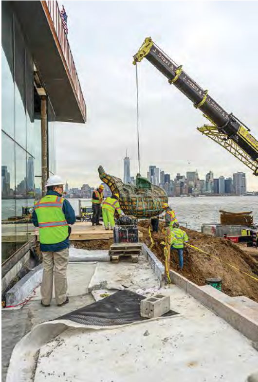
CLOCKWISE FROM ABOVE Ahead of the glass walls, the torch was craned into the museum in three pieces.
