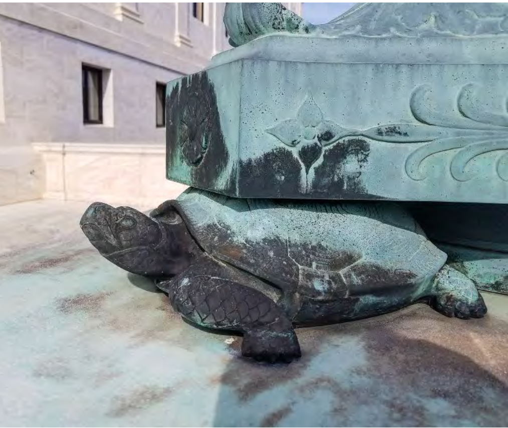
BELOW Copper stains on marble due to the base of the lamp, which sits on the marble.
