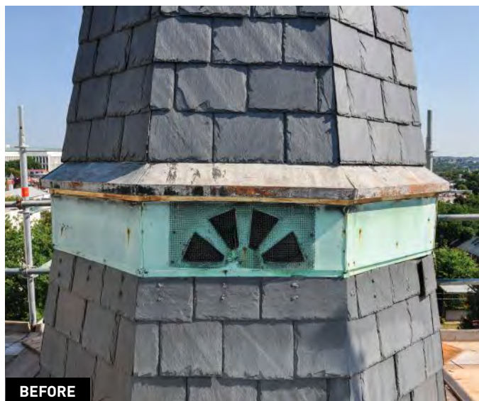
ABOVE The main tower of Mark's Episcopal Church in Washington, D.C., had four turrets that were extensively repaired and restored by the Aeon Preservation team. This entailed rebuilding wooden framing, new copper roofing and cladding, fabrication of new decorative stones, and rebuilding large sections of masonry.
