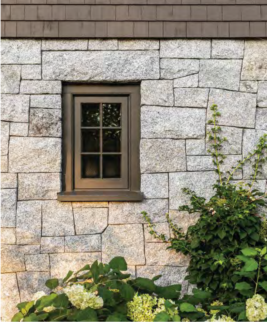
ABOVE AND RIGHT Cut-granite blocks were used for some of the structures' walls.
