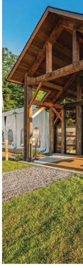
What makes timber framing appealing for modern buildings is not only the way it can span open space but also the character of natural wood and the evident structure itself. "One of the cool things about this particular building is that the central ring that forms the primary structure is essentially a parallel chord truss, a bridge truss. You can see how it kind of runs around in the middle
