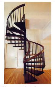
This custom 61/2-ft.-diameter stair with oak treads and open risers was manufactured by Stairways.
