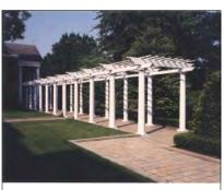
This pergola from Chadsworth was fabricated from cellular-PVC beams and rafters and PolyStone support columns.
