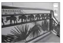
This elephant motif railing was created by **Robinson Iron** using water-jet-cutting technology.
