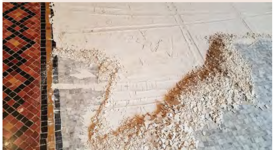
ABOVE Mosaic stone tile floor with poultice partially in place. The brown discoloration of the white diatomaceous earth is the removed dust and dirt, which was carried onto the floor by a roof leak. To the left is dried poultice partially removed from grey tile. To the right is exposed tile that was already rinsed.
