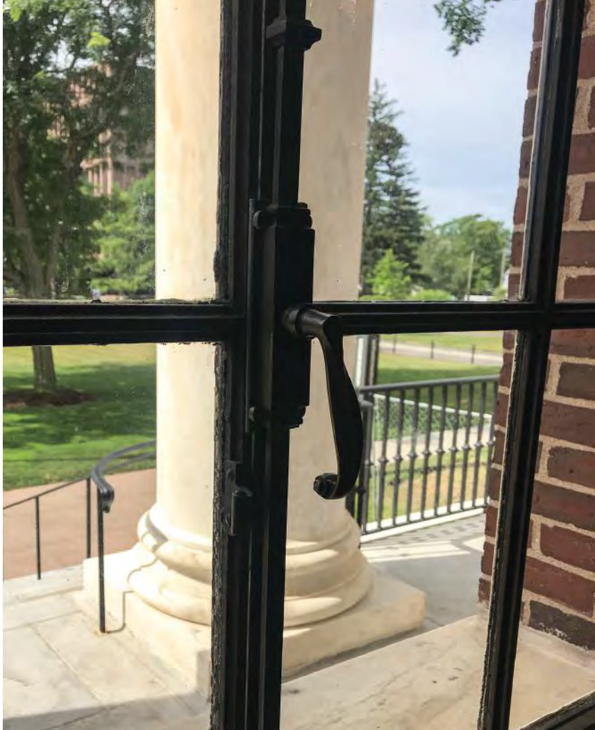
The Olin Library was designed by the firm of McKim, Mead & White, built in 1925–27. The steel windows (shown above) were in much needed repair, allowing free ingress of water and air; the brass hardware was tarnished black. You can see how the restoration of the windows brought the library back to life below.
