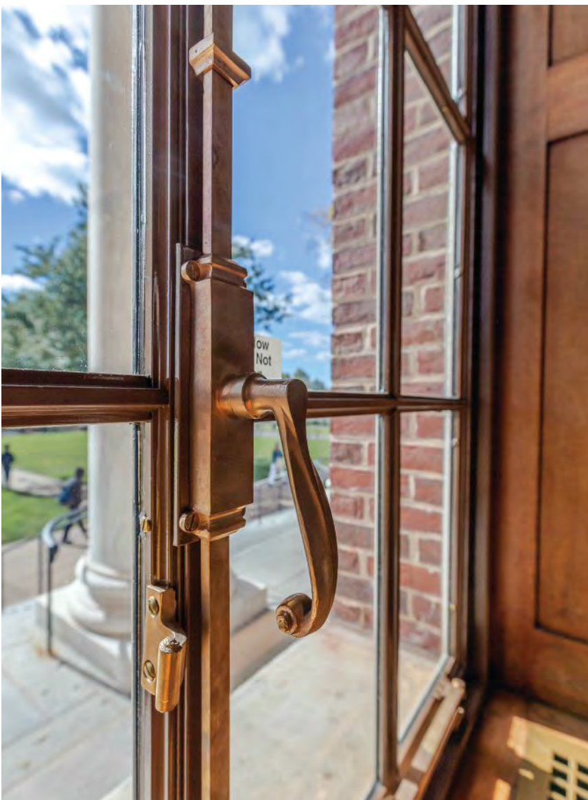
The Olin Library was designed by the firm of McKim, Mead & White, built in 1925–27. The steel windows (shown above) were in much needed repair, allowing free ingress of water and air; the brass hardware was tarnished black. You can see how the restoration of the windows brought the library back to life below.
