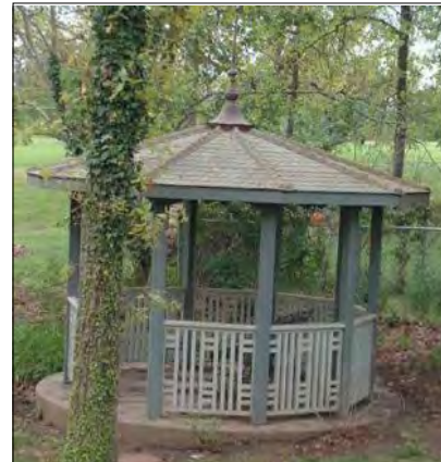
This gazebo features W.F. Norman's Style "A" shingles with its continuous hip finish and a custom-made finial on top.
