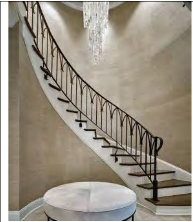
This custom designed, hand forged wrought iron staircase railing by Heritage Metalworks is intricately assembled, featuring Gothic arches and finished with a hammered texture. (Photo by Don Pearse Photography, Inc.)
