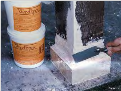
WoodEpox from Abatron can be used to repair wood elements.
