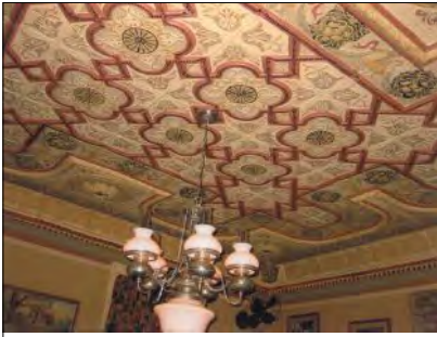
This Oriental-style ceiling was created using pressed-tin panels from W.F. Norman Corp.
