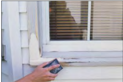
Abatron's LiquidWood restoration system regenerates and waterproofs dried out or spongy wood.
