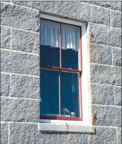
Architectural Components restored the double-hung windows to match the brick molding detail for the Customs House Maritime Museum in Newburyport, MA.
