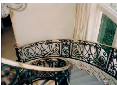
This forged-iron railing and polished-bronze cap rail were designed, fabricated, finished and installed by Wiemann Metalcraft .
