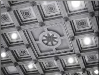
NIKO fabricated and installed these pressed-metal coffers.
