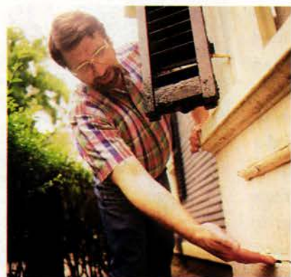
ABOVE: Anywhere water can collect, you're likely to find rot, says Norm, who found plenty around the trim on the bay window. BELOW: Although the house has no storm windows and ice must form easily on the inside in winter, Norm found almost no rot in the mullions and sash.
