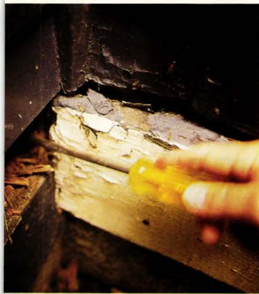
Obvious rot in trim and siding usually signals even more extensive trouble inside the wall.
