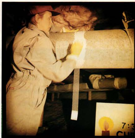
In homes with forced-air heating (and/or central air conditioning), leaky ducts can cut the system's efficiency by 25 percent or more. Above left: Helen Lugano butters a joint with RCD #6, a water-based, fiber-reinforced mastic. Then she wraps it with mesh-type drywall tape, finishing with another layer of mastic. Above right: Duct insulation is variously sized to fit around standard ducts. Seams are closed with reinforced foil tape.
