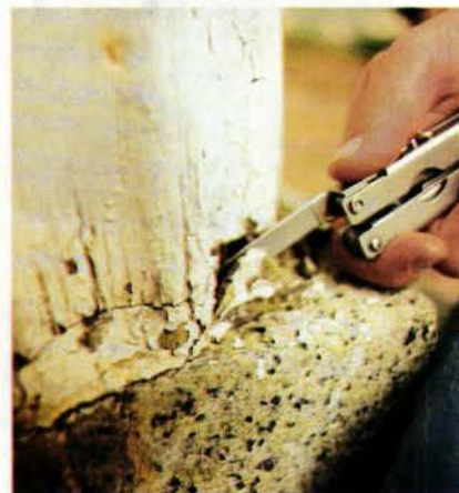
Steve's Multi-Plier detects rot at the base of a column on the front porch.
