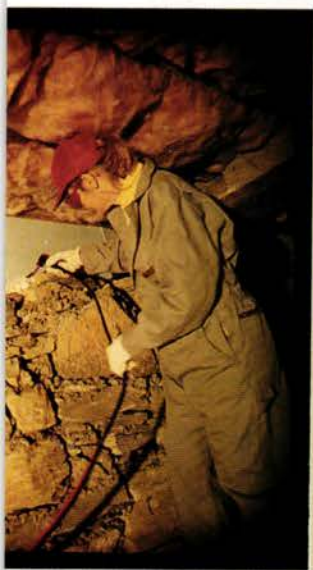
Lugano seals gaps wider than \frac{3}{8} of an inch with polyurethane foam . He pokes the tube into the opening; the foam expands inside.
