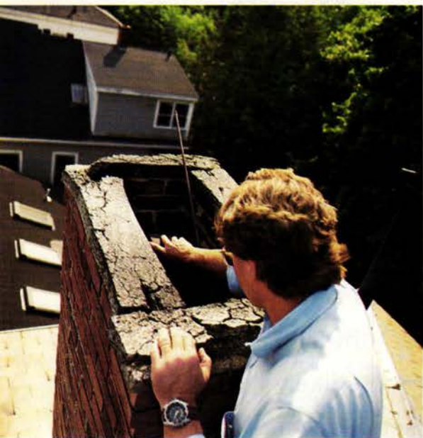
Steve checks loose and crumbling mortar work atop a chimney on the oldest part of the house.
