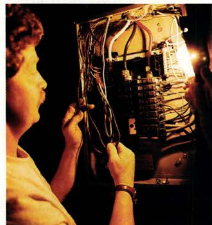
The main circuit-breaker box is the first stop on a thorough examination of home electrics.
