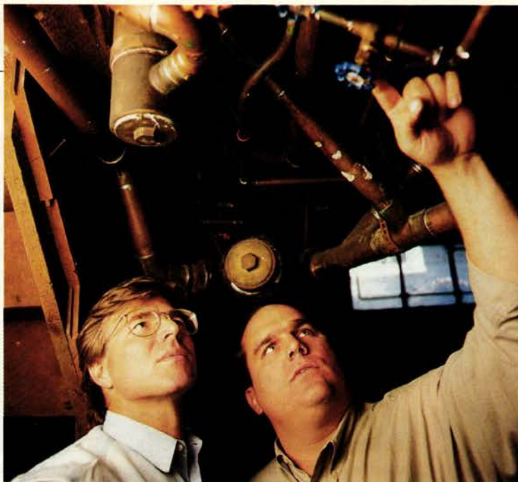
This, Richard tells Steve, is a plumbing nightmare: a jumble of unsupported pipes made of several different materials, arranged in patterns that appear to defy logic.
