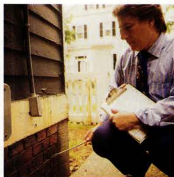
Brick is not an ideal foundation material, and on the Victorian addition it needs to be repointed.
