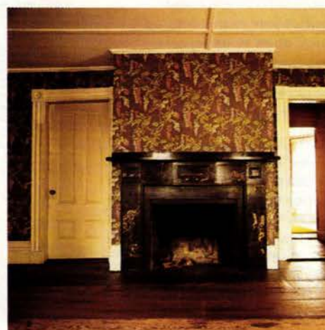
Sagging door frames next to a fireplace indicate uneven settling problems.
