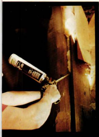
Lugano seals gaps wider than \frac{3}{8} of an inch with polyurethane foam . He pokes the tube into the opening; the foam expands inside.
