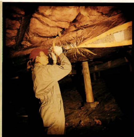
In homes with forced-air heating (and/or central air conditioning), leaky ducts can cut the system's efficiency by 25 percent or more. Above left: Helen Lugano butters a joint with RCD #6, a water-based, fiber-reinforced mastic. Then she wraps it with mesh-type drywall tape, finishing with another layer of mastic. Above right: Duct insulation is variously sized to fit around standard ducts. Seams are closed with reinforced foil tape.
