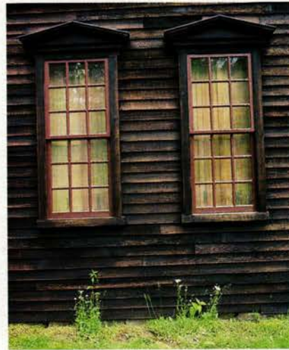
When exteriors were painted, trim came first. Venetian red protects sash at the 1743 Sheldon-Hawks house.
