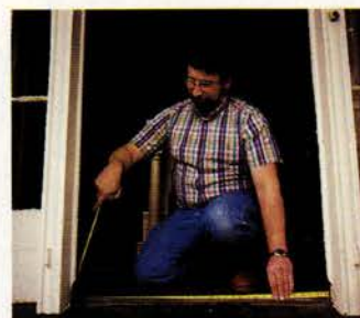
ABOVE: Norm snugs blade into doorway. BELOW: Length of flat tape plus estimate of gap equals total: 34 1/2 inches.
