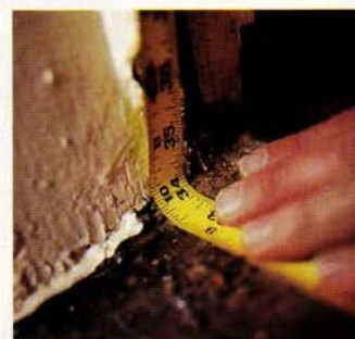
ABOVE: Norm snugs blade into doorway. BELOW: Length of flat tape plus estimate of gap equals total: 34 1/2 inches.
