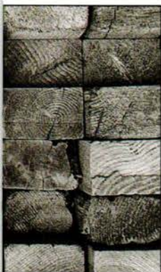
Cribbing timber is ready for stacking beneath the house.
