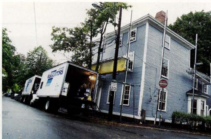
LEFT: Insulation day at the Guinees'. The chemicals and machinery stay on the trucks; only the spray hoses go inside. BELOW: Richard Trethewey and heating contractors Richard and Brian Bilo wrangle the new boiler into the basement.
