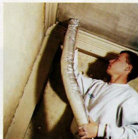
With a helper pulling from above, he feeds the duct up into the attic. If needed, additional lengths can be coupled on up there.
