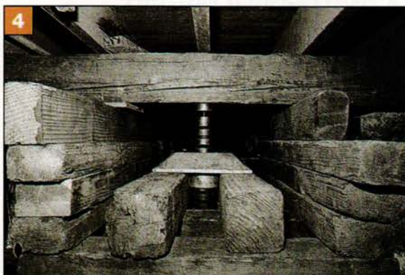
Hydraulic jacks (13 were used here) hoist the house 1 foot at a time. Cribbing is stacked around the jacks to support the house, then the jacks are reset to lift the house another foot.
