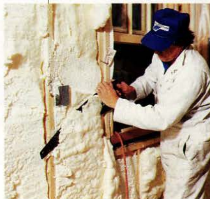
ABOVE: Open wall and roof framing is quickly filled in one or two passes. There's no need for roof vents because water vapor can't pass through the foam. LEFT: Minutes after the foam is applied, John Lojek trims off the excess with a handsaw. Trimmings don't go to waste: They're chopped up and used as loose-fill insulation in attic floors.
