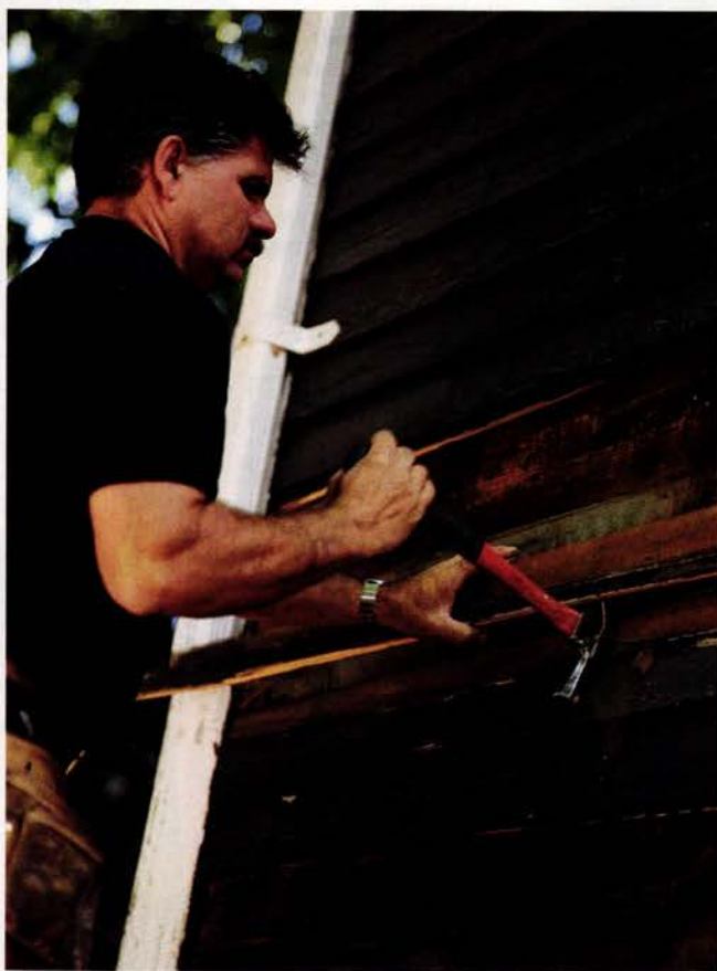
It took some getting used to, but now Tom Silva is crazy about this Yamaguchi with a long bent neck and extended handle. "It has extraordinary balance," he says, "and the long handle lets you get some beef into it for driving nails."
