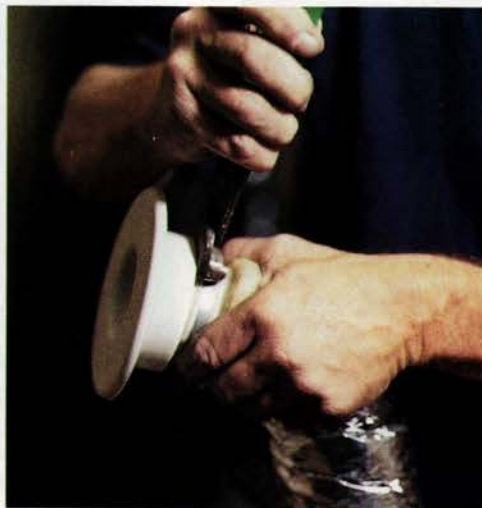
The outlet finish plate slips easily into the end of the duct. It is then clamped tightly to prevent possible air leaks.
