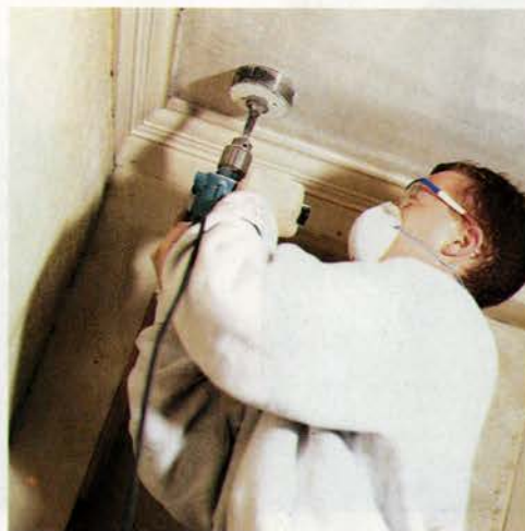
To bring a warm air outlet into a room, Brian Bilo starts by drilling a 4-inch hole through the plaster and lath in the ceiling.
