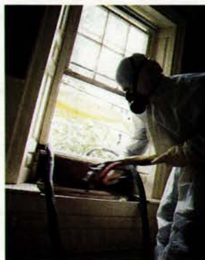
Built-in window seats at the Guinees' house are lovely details but also a big source of drafts and heat loss. With a few pulls of the trigger, Gustavo Nadales plugs the leaks and fills the cavity. It's a case of giving up a little storage space and gaining big energy savings.
