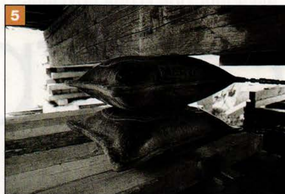
Because of the size of the Coen house, the jacks were augmented with air bags. The jacks and air bags must be synchronized to move at exactly the same pace. If one jack or airbag is off by as little as an inch, the house will pitch and corkscrew.
