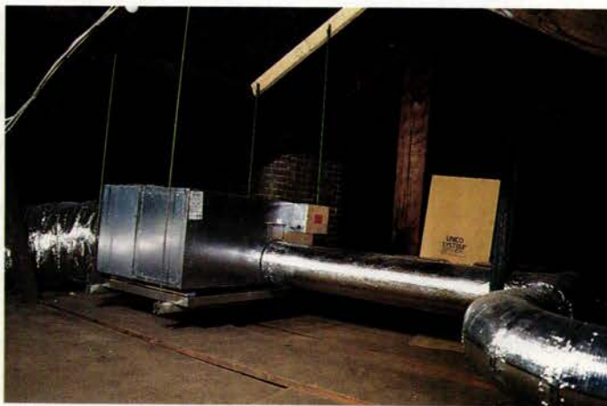
The Unico fan/coil—which houses the heat exchanger and blower in a sheet-metal box—sits in a drain pan suspended from the rafters. This arrangement, with the addition of a few rubber pads, minimizes vibrations that would become noise in downstairs rooms. If the Guinees ever want central air conditioning, a cooling module can be added with a simple system of clamps and gaskets.
