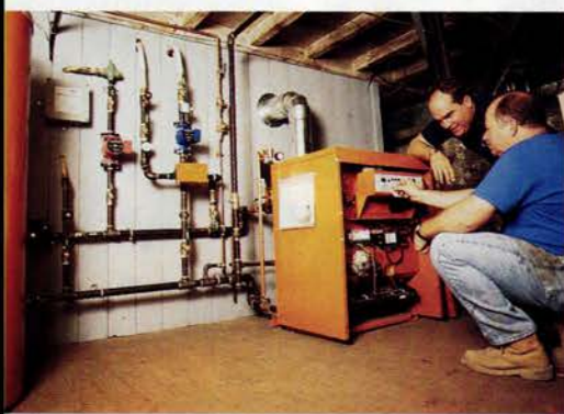
The two Richards, Trethewey and Bilo, ready the new microprocessor-controlled boiler for three functions: warm air, warm floors and hot water.
