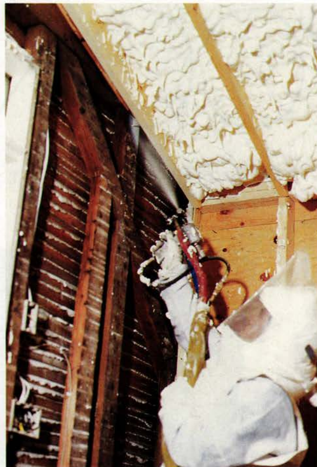
ABOVE: Open wall and roof framing is quickly filled in one or two passes. There's no need for roof vents because water vapor can't pass through the foam. LEFT: Minutes after the foam is applied, John Lojek trims off the excess with a handsaw. Trimmings don't go to waste: They're chopped up and used as loose-fill insulation in attic floors.
