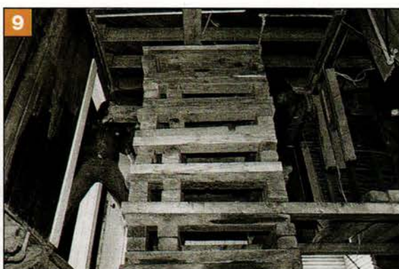
The stack of cribbing grows as the house rises. The house remains on the cribbing for two months while a new foundation is poured and wooden piers are set. Then A.C. Hanna returns and lowers the structure onto the new foundation.
