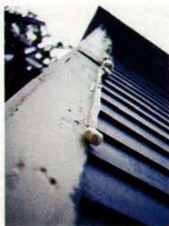
Foam that has expanded all the way to the outside is proof positive that it can seal otherwise inaccessible air leaks.
