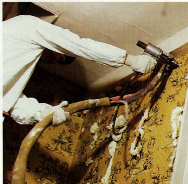
To fill a wall, Ted Franklin presses his gun into predrilled 1-inch holes. He starts at the midpoint and finishes near the top. Overflowing foam tells him the cavity is filled.
