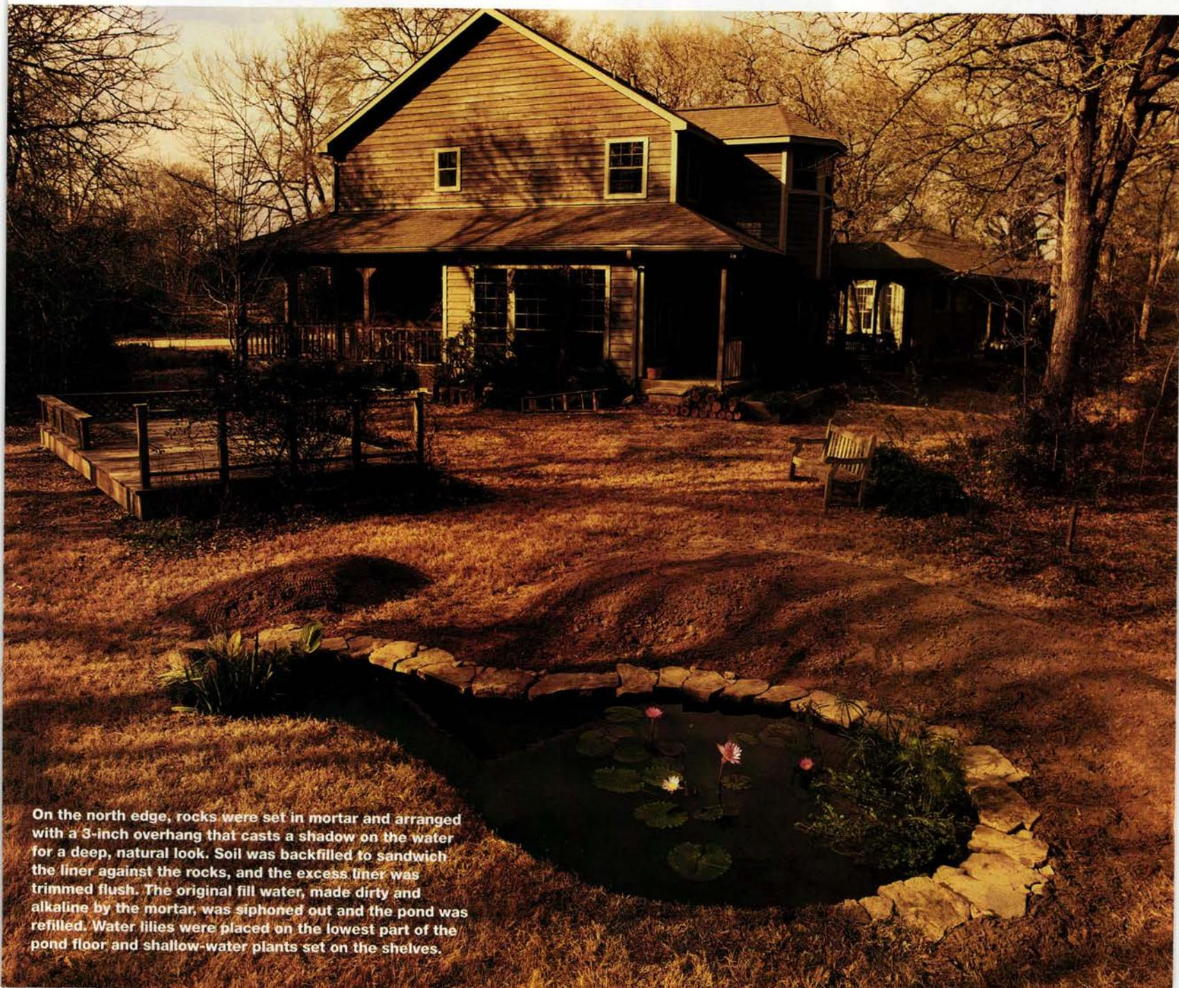
On the north edge, rocks were set in mortar and arranged with a 3-inch overhang that casts a shadow on the water for a deep, natural look. Soil was backfilled to sandwich the liner against the rocks, and the excess liner was trimmed flush. The original fill water, made dirty and alkaline by the mortar, was siphoned out and the pond was refilled. Water lilies were placed on the lowest part of the pond floor and shallow-water plants set on the shelves.
