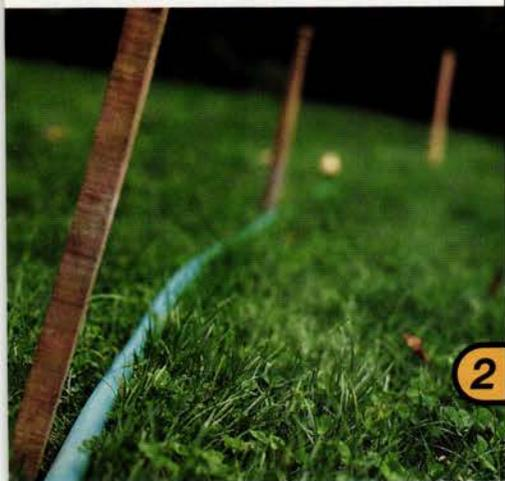
2. Before the path is dug, 1x2 stakes are driven into the ground to mark the borders. Spruce 1x3 strapping will be fastened to the stakes with drywall screws to define the exact edges of the 48-inch-wide walkway.
