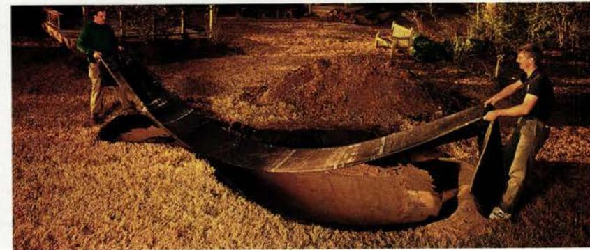
Matting around the sides of the pond and sand on the bottom keep any remaining sharp stones and roots from damaging the liner. A synthetic feltlike underlayment fabric was cut into panels to fit the sides. (Old carpet can also be used.) Liners come in many sizes and are made from materials such as inexpensive PVC or more costly, longer-lasting rubber. Thicker liners last longer—up to 50 years.
