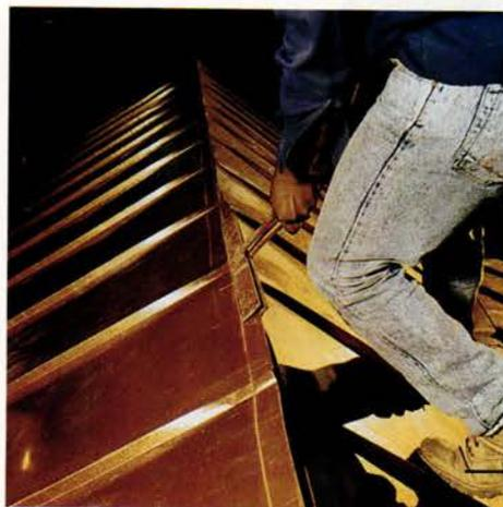
**The ridge cap was created by hand.** Eighteen-inch tongs were used to push the metal from each side of the dormer into a standing position. The pieces were folded over twice, much like the seams between panels. To form a crisp edge, the seam was flattened with a 16-ounce sheet-metal hammer. The ridge assembly is airtight as well as watertight, so vents must be installed every 12 inches along the soffit for attic ventilation.
