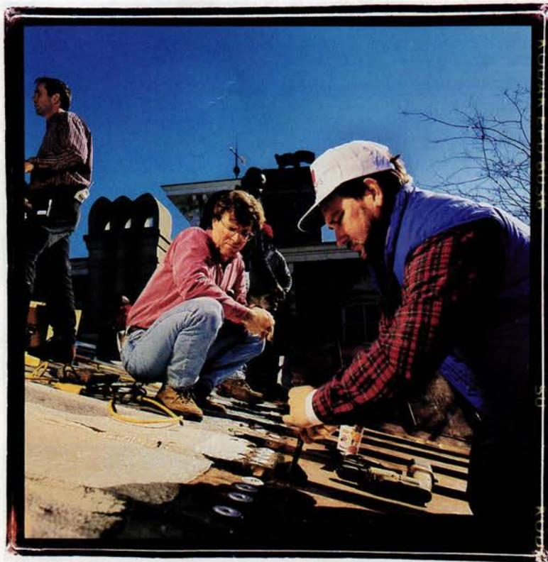
**As Steve watches, roofing contractor Jeffrey Lancaster seals the seam between the new roof and the old.**
