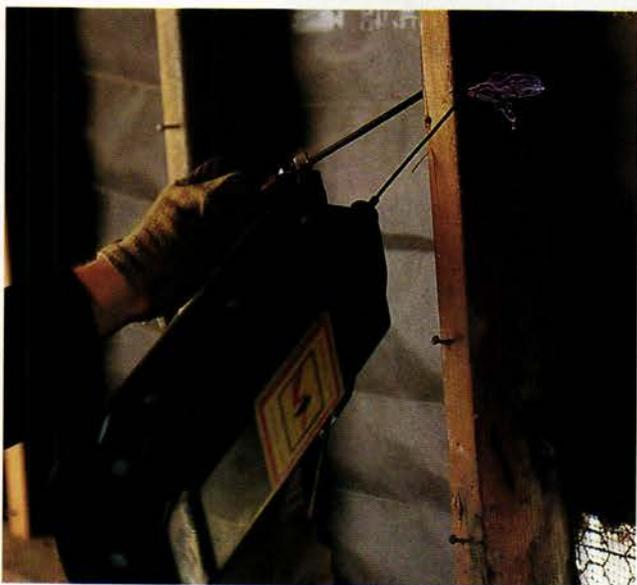
Fingers of blue light dart across a 2x4 under a house in Castro Valley, California, as Todd Maitlen of Northwest Termite Control uses the Electro-Gun to search out drywood termites. The gun shoots pulses of electricity at a low current (about .5 amp), high voltage (90,000 volts) and high frequency (60,000 cycles). When the current hits a termite tunnel, it jumps from the gun, through the wood, to a screwdriver that acts as a ground. Termites in its path are killed.
