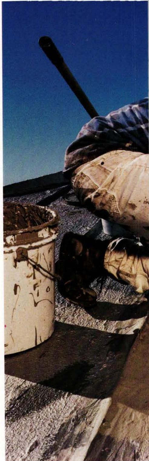
ABOVE: AcryMax can be used with or without the polyester reinforcing mesh. The mesh gives the acrylic coating additional strength and, in effect, holds the roof together. The coating can be ordered in just about any color. On the Fleming house, AcryMax was installed by contractors, but homeowners can do the work themselves—as long as they aren't afraid of heights.
