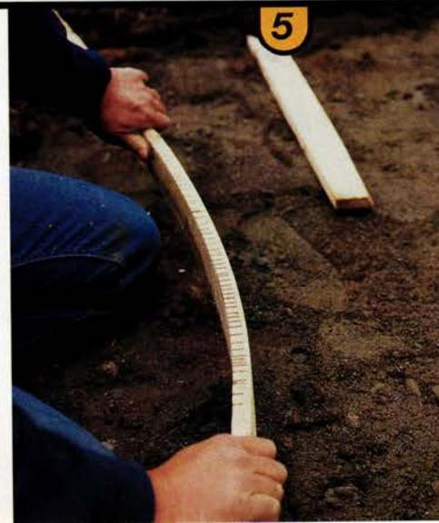
5. The spruce boards that control the sides and width of the walkway are bent into curves by kerfing them—sawing partway through across the grain every half inch or so. Boards should be securely placed so the width of the walk varies by less than 1/4 inch.
