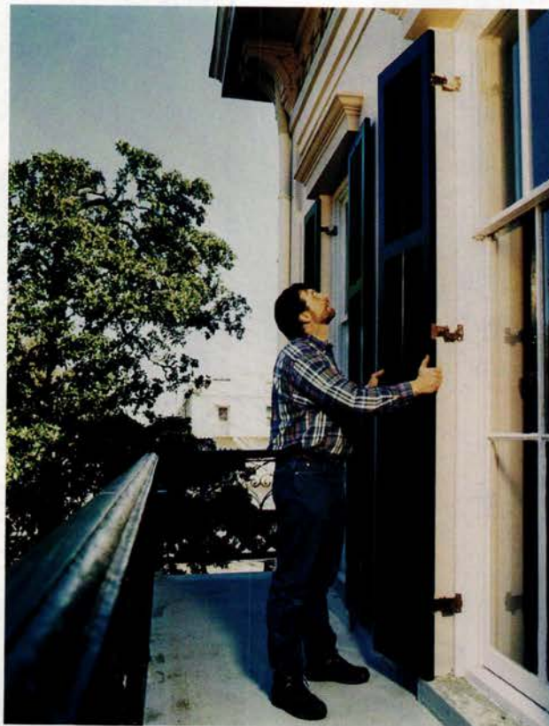
Norm Abram installs a shutter on the Savannah project house. The hinges are in the proper position: inside the window casing, not beside it.
