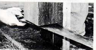
10" rotted bottoms of these load-bearing columns...
