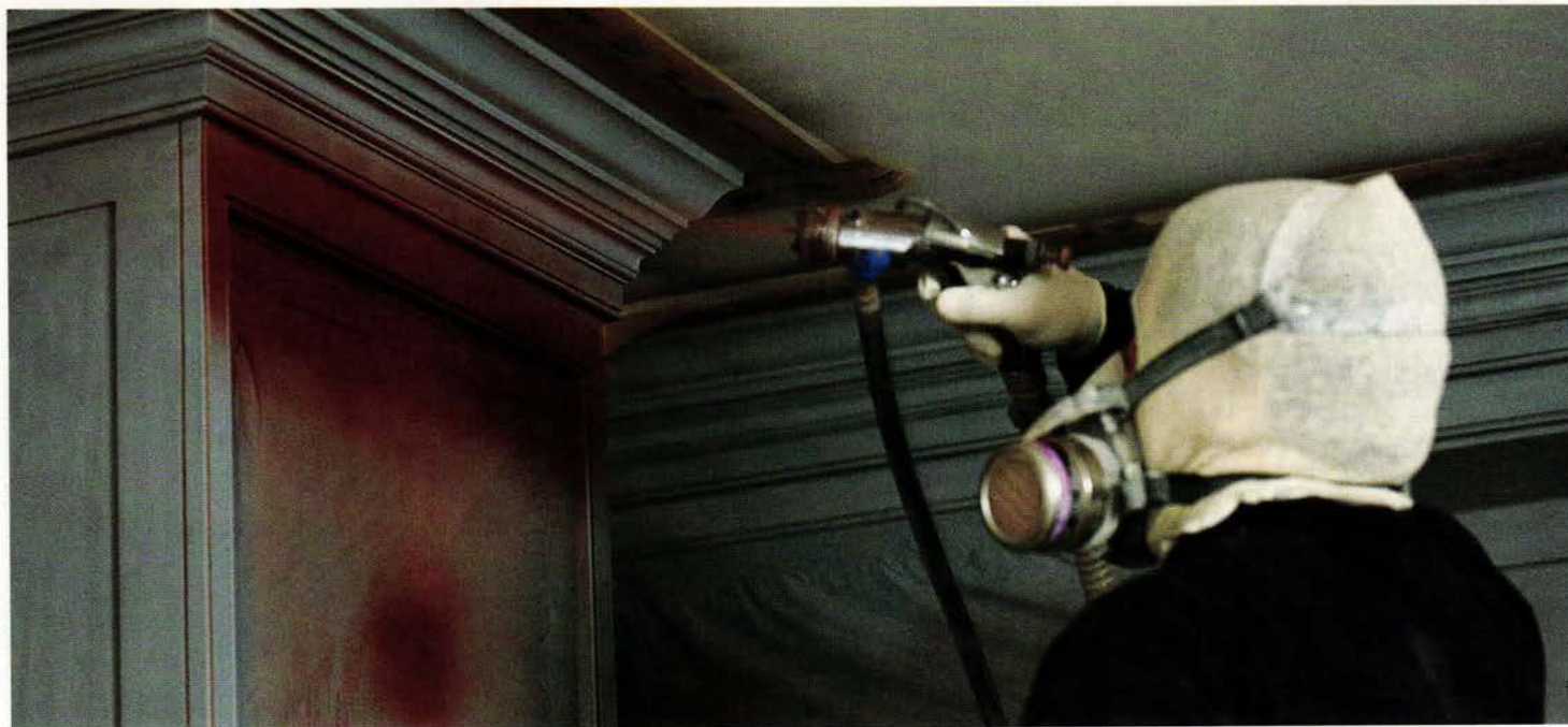
With skin, lungs and ceiling protected, Dee spray-paints crown moldings with his HVLP gun. For fine work, he restricts paint flow. "You can just about turn the gun into an airbrush," he says, referring to an artist's tool that paints with pinpoint control.
