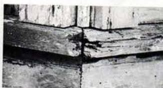
This rotted - and irreplaceable - woodwork...
