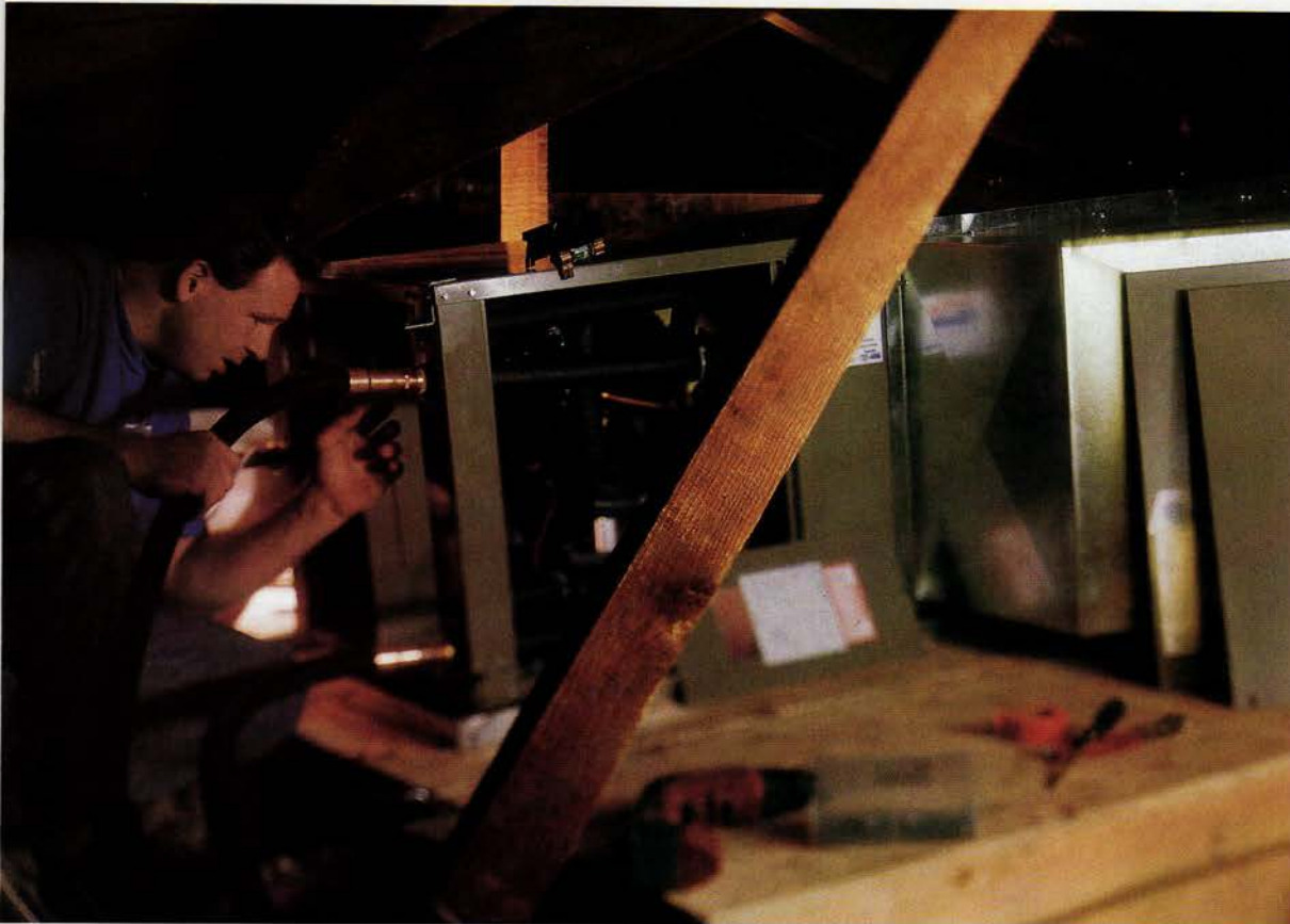
Tubing that connects the flow center to the attic compressor unit was run through what used to serve as the laundry chute. The unit fits snugly beneath the roof rafters.
