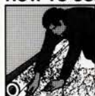
1. Cut fiberglass mat 2" longer than height.
