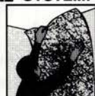
3. Apply fiberglass mat to wet surface.
