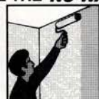
2. Apply saturant to area to be covered.
