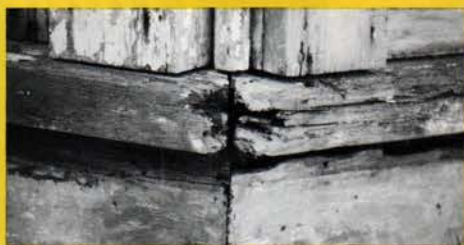
This rotted – and irreplaceable – woodwork...
