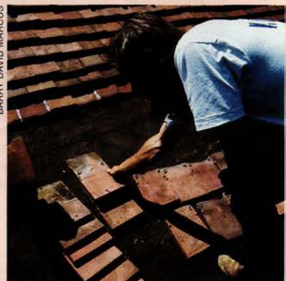
Clay tiles aren't waterproof. They work by protecting an underlying waterproof membrane from damaging ultraviolet light.
