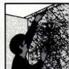
4. Trim excess mat where wall meets ceiling.
