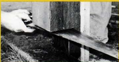
10" rotted bottoms of these load-bearing columns...
