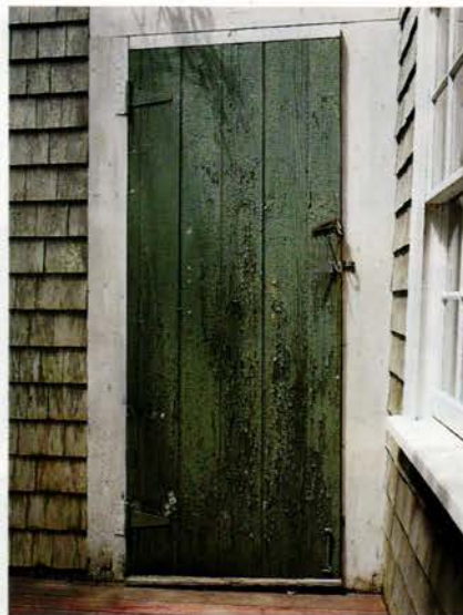
A batten door, on what's known as The Little Red House, is built like a ship's hatch.
