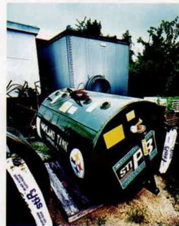
The STIP3 tank has a sacrificial zinc anode hanging from it like a white buoy.
