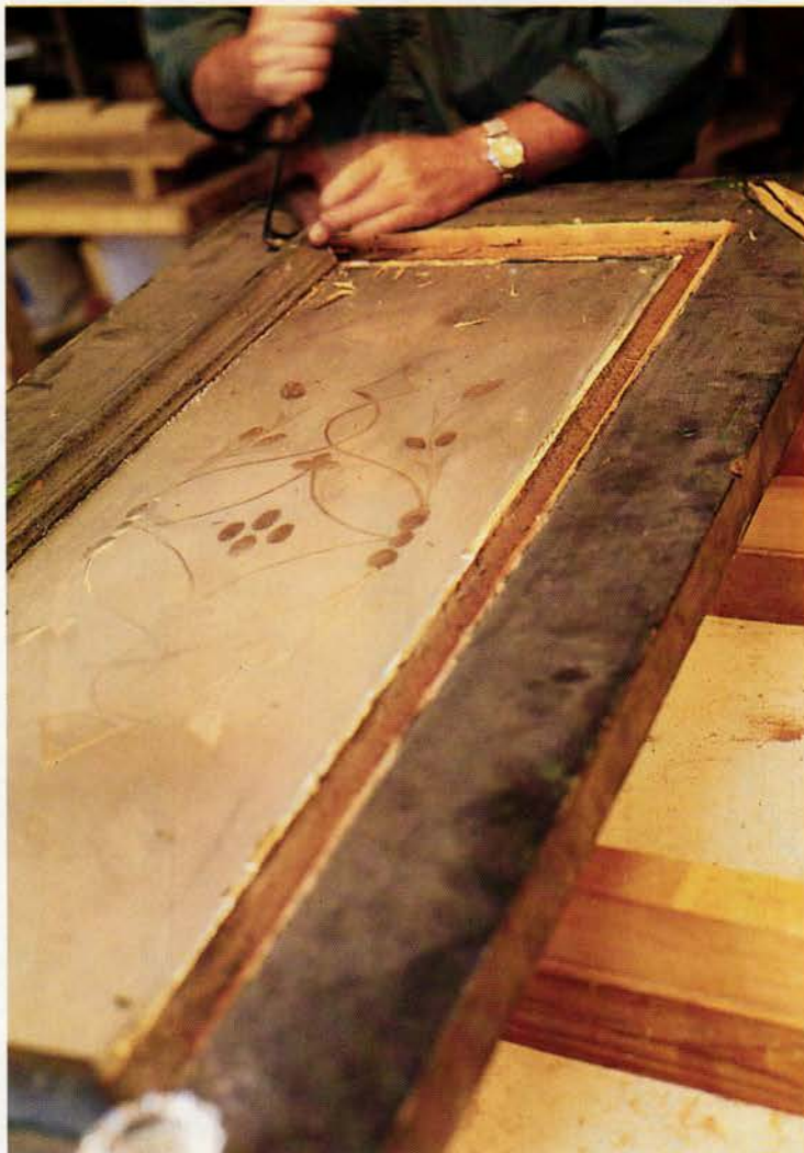
ABOVE: Tension is high in Bruce Killen's shop as moldings are pried off to free the surviving cut-glass pane. RIGHT: Cracks were filled with epoxy before the doors were cranked tight.
