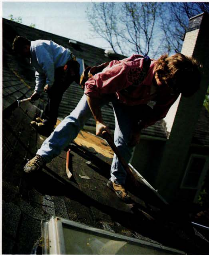
Tom Silva and Steve Thomas started by stripping off the shingles and roofing felt. They also removed the gutter so it wouldn't be damaged during the project.
