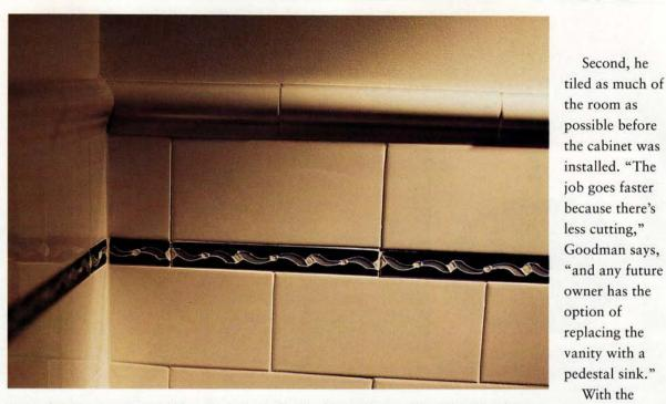
Symmetrical, mirror-image tile work is the hallmark of a meticulous tile-setter. Goodman used his diamond-bladed bandsaw to miter the bullnose tiles capping the wainscot.
