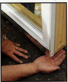
H2O test If joints aren't sealed, moisture can rot a wood window. To check for leakage, Tom taped a dam across the Haggers' new window and poured in water. It leaked, so he caulked the joint.
