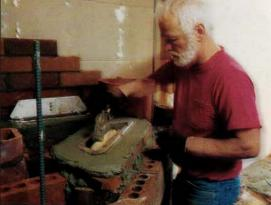
Next Buckley attaches stainless-steel dampers that have been custommade to fit the narrow opening of a Rumford's throat. A wide mortar-andbrick bed encases the throat.
