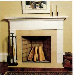
ABOVE: Buckley sets a clay flue liner in place above a twopiece triangular clay smoke chamber that rests atop the throat. LEFT: The finished fireplace awaits its inaugural blaze. The thin black metal band surrounding the firebox opening is a door frame, shown here without glass doors. Buckley likes to set his logs tepee-style against the fireback to take advantage of the tall fireplace. A taller fire also enhances efficiency and emission.
