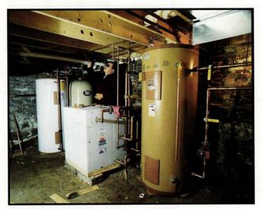
In the cellar, the cube-shaped unit is the ground source heat pump. It takes 51-degree water from a backyard well and extracts warmth from it to heat the house. In summer, the process is reversed to provide air-conditioning.
