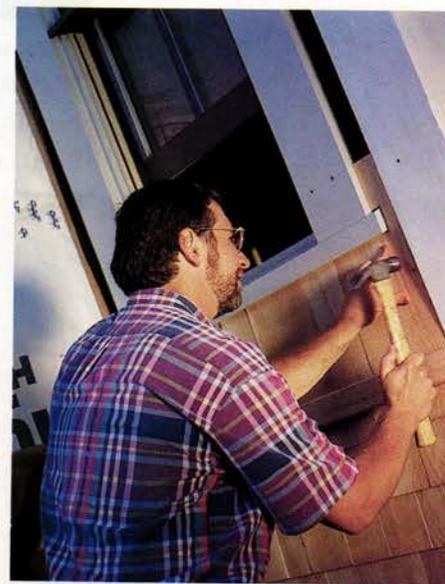
For a weathertight fit around windows, Norm Abram notches the shingles next to the sill horns.
