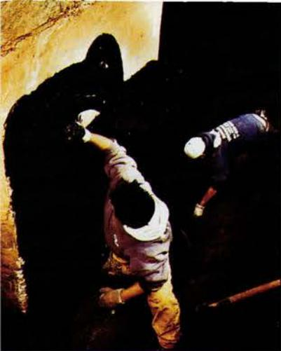
**Instead of using foundation tar, a worker seals the exposed wall by quickly smearing on a layer of 60-mil-thick fibered cement, similar to roofing cement.**
