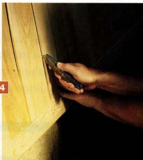
**Norm shingles from either end of a course toward the center. He gets a tight fit between the last pair by overlapping them, then scoring the one underneath with a utility knife and snapping off the waste.**
