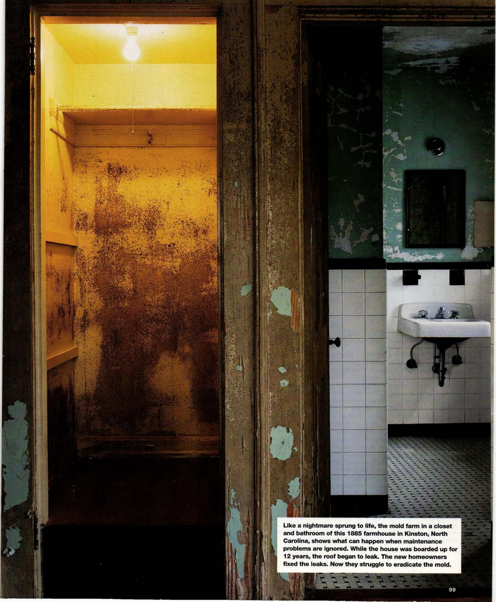
Like a nightmare sprung to life, the mold farm in a closet and bathroom of this 1885 farmhouse in Kinston, North Carolina, shows what can happen when maintenance problems are ignored. While the house was boarded up for 12 years, the roof began to leak. The new homeowners fixed the leaks. Now they struggle to eradicate the mold.
