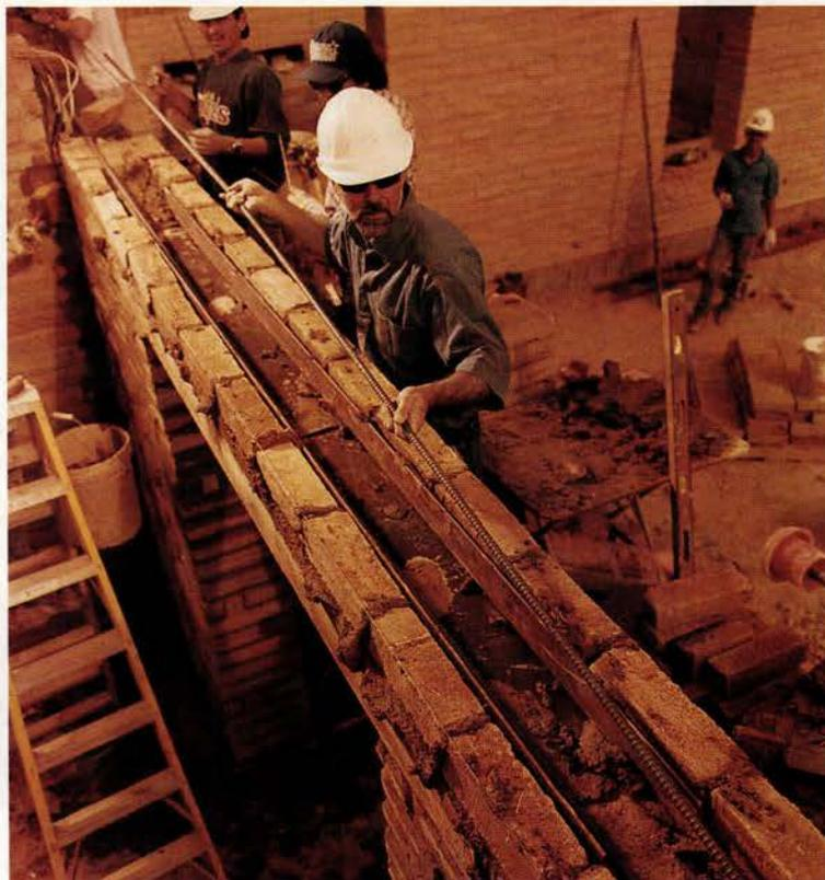
Buckets of concrete are poured into the cavity to form a steel-reinforced, 8-by-8-inch concrete beam. A similar continuous beam (minus the angle iron) is poured at the top of every wall in the house.
