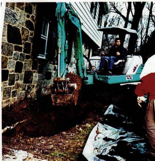
Careful to avoid smashing the stone facade or ripping into lines for water and natural gas, waterproofing expert Dean Maiorano maneuvers an excavator across the front of McMoran's house and digs a trough down to the footings.
