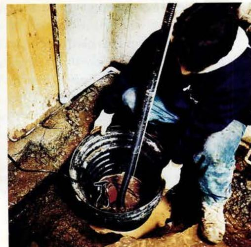
below the concrete slab, middle. Interior systems require a gravity feed or a sump pump, which is installed in a shallow well, bottom left. Once the pipe is placed in the trench and covered with gravel, below, a plastic vapor barrier, bottom right, is laid on top and then patched with cement. "We've had lots of rain since," Angley says, "but it's been dry as a bone."
