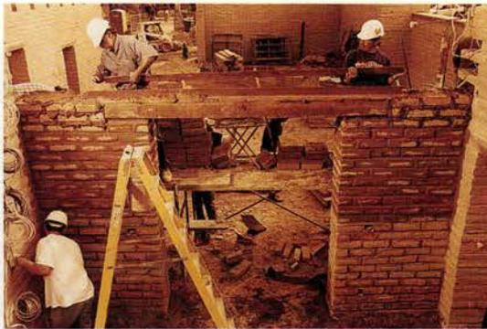
Small adobe veneer bricks are laid on either side of the angle irons. This creates a form for pouring and concealing the concrete beam.
