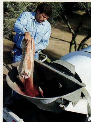
John Carson pours colorant in a concrete truck's hopper. It must churn for 30 minutes to ensure thorough mixing.
