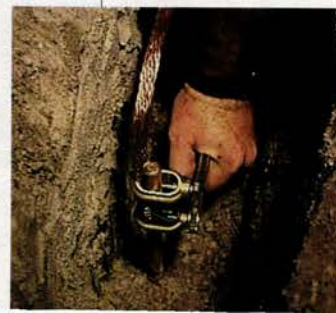
Ron Miller drives a 10-foot ground rod at least 2 feet from an exterior wall, above, and then attaches the cable to the rod, below.
