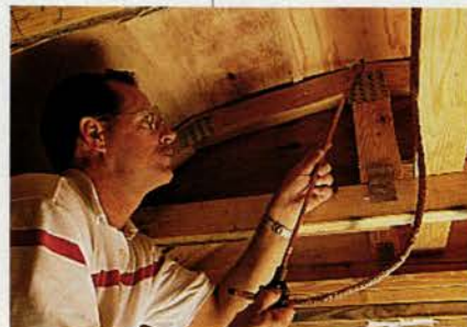
In the rafters, he identifies the spot where he will put the terminal through the roof.
