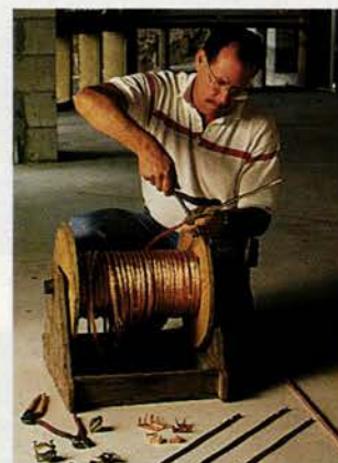
Installer David Vann clamps an air terminal to a length of copper cable.
