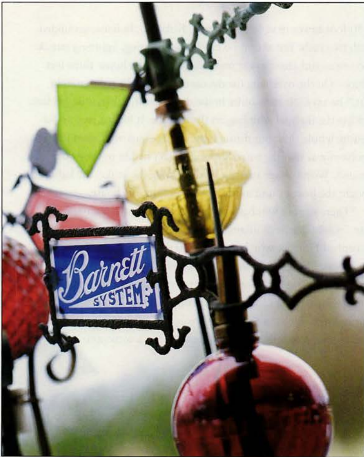
Early lightning rod makers took to adorning their sky stakes with survivable materials like glass, which wouldn't conduct the jolt.
