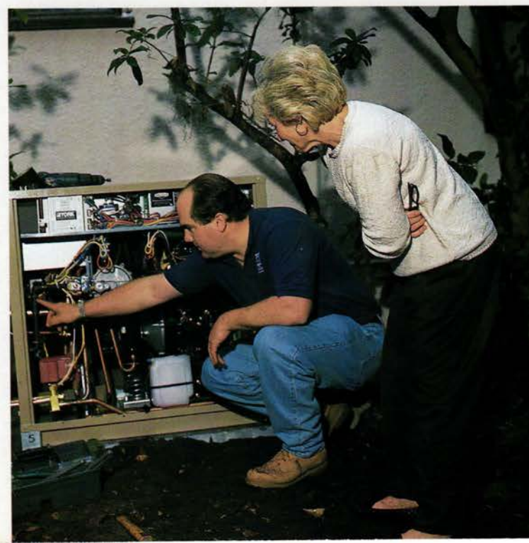
Before the Triathlon was fired up, Richard showed the engine, compressor and condenser to homeowner Sandy Kirk. “Unlike other heat-pump or air-conditioning units,” he says, “the Triathlon has all of its serviceable parts accessible through one panel.”
