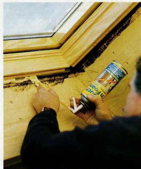
Urethane foam seals the gap between frame and skylight, preventing water from collecting on the flashing's underside. "A lot of people think their skylights are leaking," Tom says, "but they're really condensing on the inside."
