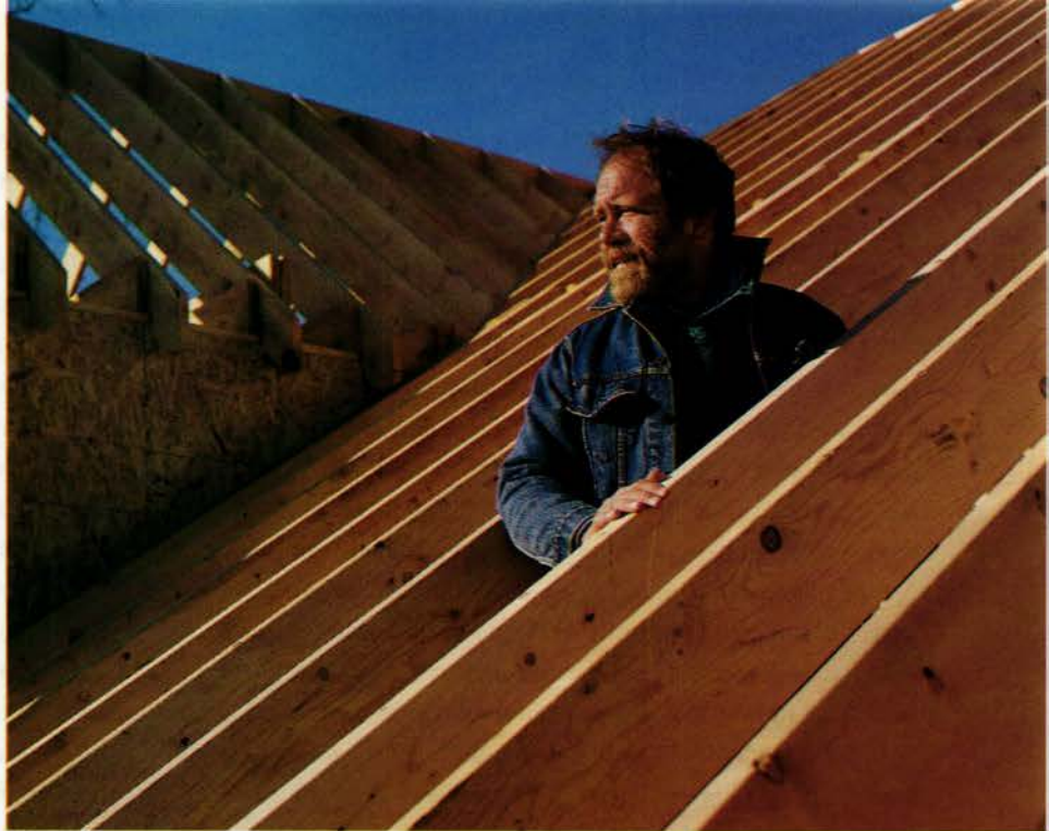
Perched on the ceiling joists of a house in Columbus, Reade admires the precision workmanship in the hand-cut 2x12 rafters. "This is called rough carpentry, but that's just a designation. There's nothing rough about it."
