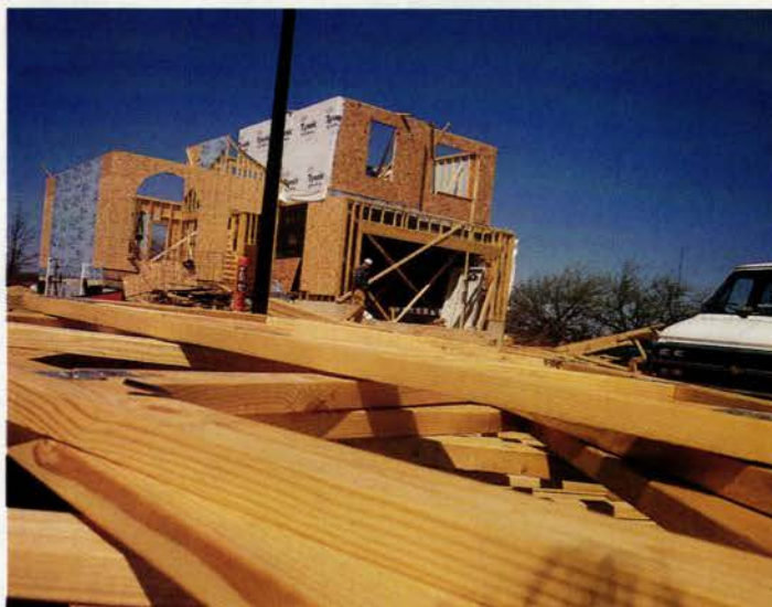
Trusses lay stacked and ready to be lifted by crane onto the roof of a newly framed tract house, one of the 1.35 million wood homes built every year in the United States. On average, 15,000 board feet of lumber is used in the construction of a single house.
