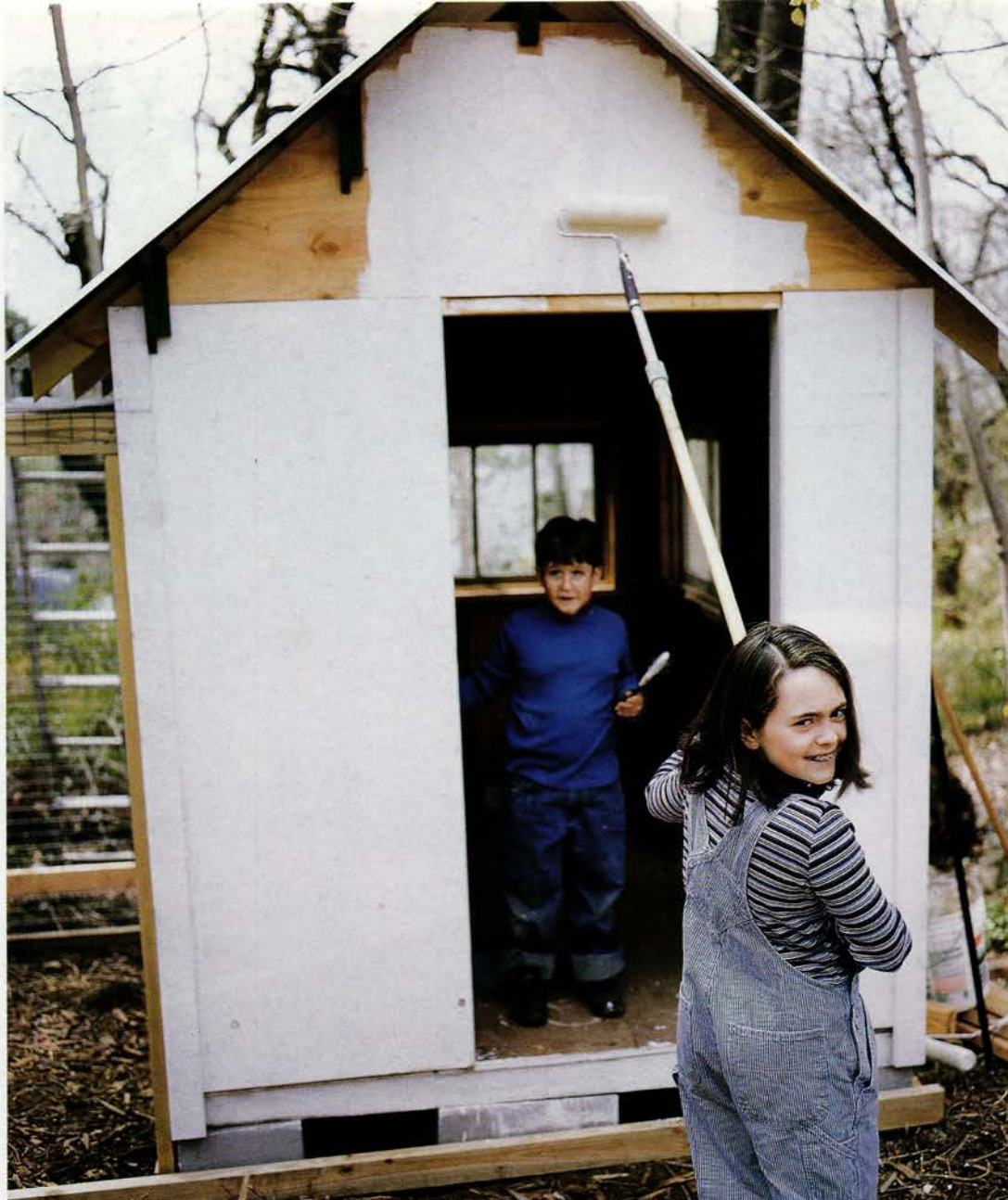
Jake DeMichele supervises as Olivia Carrano finishes painting the coop's half-inch plywood siding. Salvaged windows bring in light, and triangular openings in the eaves provide ventilation.
