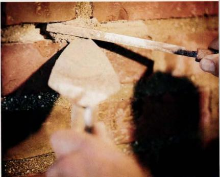
TOP: Good gutter screens let in water, keep out leaves and swing out of the way for routine maintenance. ABOVE: With a fresh application of mortar, a repointed brick wall is like new. RIGHT: The drip groove kerfed into the bottom of this windowsill stops water from finding its way behind the siding.
