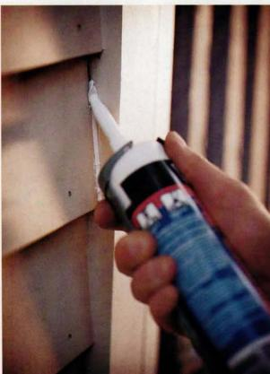
TOP: A foil-covered foam box, dogged down with straps, minimizes the heat loss through normally leaky attic hatchways. Loosen the straps, and the lightweight box moves aside for attic access. ABOVE: A paintable silicone sealant keeps air from finding its way between clapboard and corner board. To cut off another possible draft, install and caulk more blocking between the joists where they pass under the knee wall.
