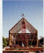
LEFT: Apprentice Jesse Grout peels away the siding of the old barn. BELOW: Project head Ken Epworth assembles the frame on the ground, using mortise and tenon joints fixed with hand-hewn pegs. "You're either an old-wood person or you're not. Some guys can't handle the splinters." TOP: Cranes hoist the bays into place on their new site.
