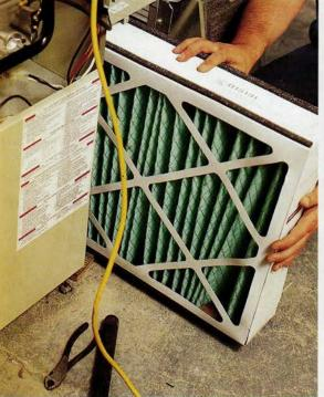
TOP: To keep it balanced, a furnace blower should be brushed and vacuumed free of gunk and dust. LEFT: An in-duct media filter cleans air far better than standard filters. BELOW: Besides adding needed moisture, a dirty humidifier can also put mildew and microorganisms into the air. Clean it often.
