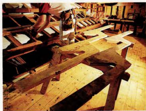
A solid aluminum replacement rafter, right, lies beside a plywood template that mimics the lightning-bolt shape of the original rafters. To minimize the possibility of damage to the roof, the carefully choreographed replacement is executed mostly with hand tools.
