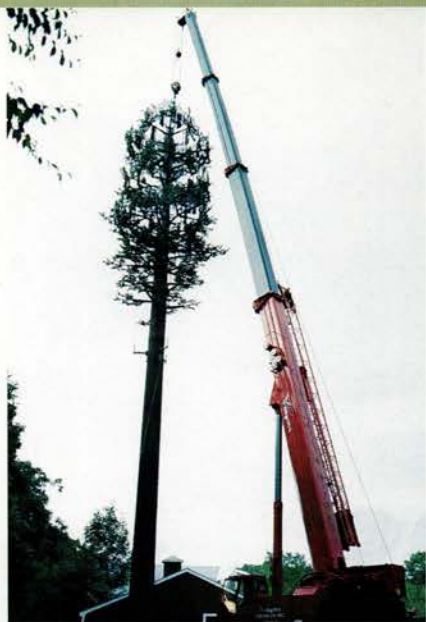
A crane lifts a camouflaged cellular-phone tower into place in Franklin Lakes, New Jersey.
