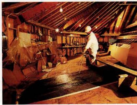
Boatbuilders from the famed Palmer-Johnson yard in Sturgeon Bay, Wisconsin, stiffen Wingspread's lower roof with 14 layers of carbon fiber glued together with waterproof epoxy, creating a lightweight laminate never previously used as a roofing material.
