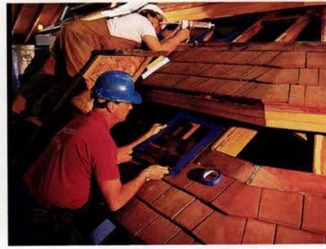
Workmen install new insulated skylights using silicone sealant to prevent leaks. The replacement clay tiles, made from molds of the water-damaged originals, are held in place by an elaborate earthquake-proof system composed of stainless steel straps and wires.
