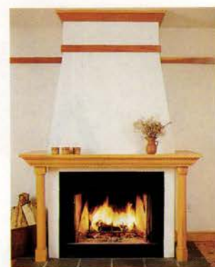
Wedlick designs many of his fireplaces, above, so the eye focuses on the space around the fire. He favors inexpensive pine moldings and drywall as well as prefabricated steel fireboxes.
