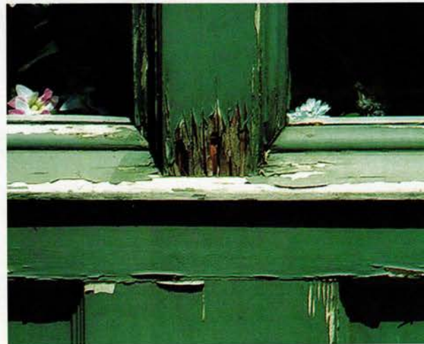
With no pre-paint preservative, rot sets in after only a year.
