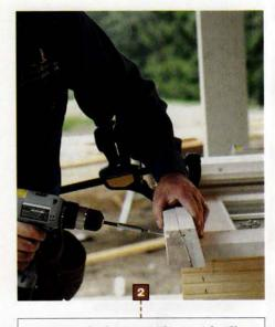
Tom can't find new windows with sills as thick as the old ones, so he orders sill extensions. First he spreads construction adhesive between sill and extension. Then he clamps them together with screws before caulking any remaining gaps. After beltsanding and painting, the glued-up sills closely match the one-piece originals.
