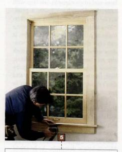
At the end of the job, Tom nails the apron beneath the stool. He sands the newly installed trim to remove mill marks. It all fits perfectly—except for the slender gaps between the side casings and the uneven wall. "I could just fill them with caulk," he says. Instead, he carefully scribe-fits strips of poplar and glues them in place.
