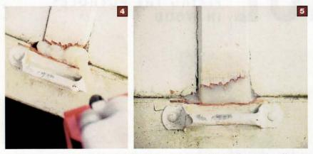
**4.** After the cavity is coated with a thin epoxy primer, it's filled with a much stiffer mix of resin and hardener squeezed from a special twin-tube caulking gun. **5.** The epoxy can be shaped and smoothed for 20 to 60 minutes, depending on the air temperature. After curing for a day or two, the patch is ready for sanding and painting.
