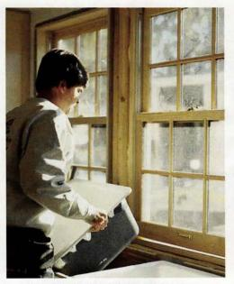
Charlie Silva drops in the sinks so they sit flush, centered above the two base cabinets. Vermont Soapstone workers can make a template for cutting the sink holes in the counter.
