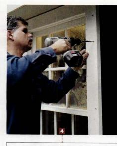
Tom affixes the window to the framing permanently with  $2^{1}/_{2}$ -in. stainless-steel screws placed 12-16 in. apart. (No screws through the sill, though.) "You want to make sure they're going into the structure of the wall, not just the sheathing," he says. Afterward, he'll either putty over the holes or leave them flush and paint the heads.
