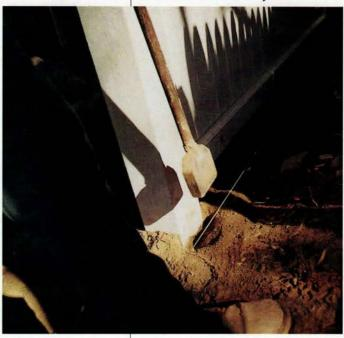
An iron tamping bar pounds the soil tightly around the post while it is held plumb. Porous soils make the best fencepost packing. About the only force that will lift a well set post is a frost heave. The fence company's one-year warranty provides for a return visit to correct such problems.
