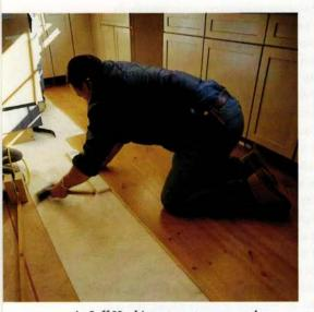
As Jeff Hoskings taps tongue-and-groove laminate floor strips into place, he uses a polyethylene block to cushion the blows.
