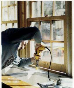
After the sink holes are made, Jim Heath of Vermont Soapstone uses a hole saw to cut out three plugs for a single-lever faucet, a sprayer and an instant hot-water dispenser.
