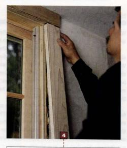
Once the stool is in place, Tom trims the rest of the window with poplar, nailing it tight to the jambs. The low ceiling forces him to install the head casing before biscuit-joining the side pieces to the head trim. (It's easier to trim the head last.) He then anchors the lower end of each side casing with a screw through the stool.
