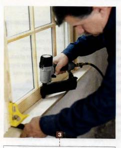
The stool, a piece of poplar 1 in. by  $3^{1/2}$  in., is long enough to project 1/2 in. beyond the edges of the side casings. With a series of scribes and cuts, Tom fits the stool within a "hair's width" of the sash; then he glues and brad-nails it to the sill at 6-in. intervals. Bracing a combination square against the frame keeps the stool level as he nails.
