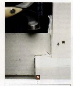
Before he nails the siding in place, Tom guns sealant between the window casing and the spline, creating one more barrier against leaks. Then he squishes the ends of the clapboards into the goop and nails them down. Shielded in this way from ultraviolet rays, the caulk should last years longer than its warrantied life span.
