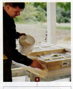
Wooden windows last longer with one moisture-repellent coat of oil-based primer on the back of the casing. It may be overkill, says Tom, but priming protects the wood from moisture exiting the house or seeping around the edge of the casing during a rainstorm. The exterior of the casing and sash was primed at the factory.
