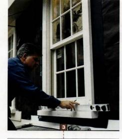
Tom's level shows that the window is slightly higher on the right, a problem he can correct either by taking it out and trimming a bit off the lower end of the right jamb or by shimming up the left jamb. Before he fastens the window to the wall, he slides both sash open and shut as a final check that everything is OK.
