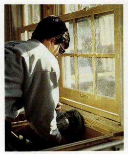
To under-mount the cast-iron sinks so they won't have a protruding lip, Tom Silva's nephew Charlie Silva shaves 1/2 in. off the top of the cabinet boxes with a plunge router.
