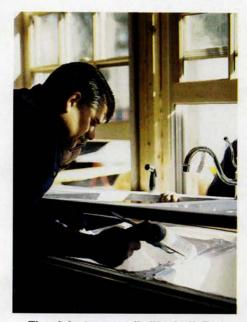
The sinks temporarily lifted off, Tom squirts silicone sealant around the perimeter to hold the counter and act as a watertight barrier between the basins and the cabinet.
