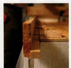
A side view of the concrete form, right, reveals how long screws anchored by small wooden blocks will prevent the walls from yielding to the pressure of wet concrete. When the form is about half filled, Mercado and Martinez, below, press lengths of galvanized steel reinforcing mesh into the concrete.
