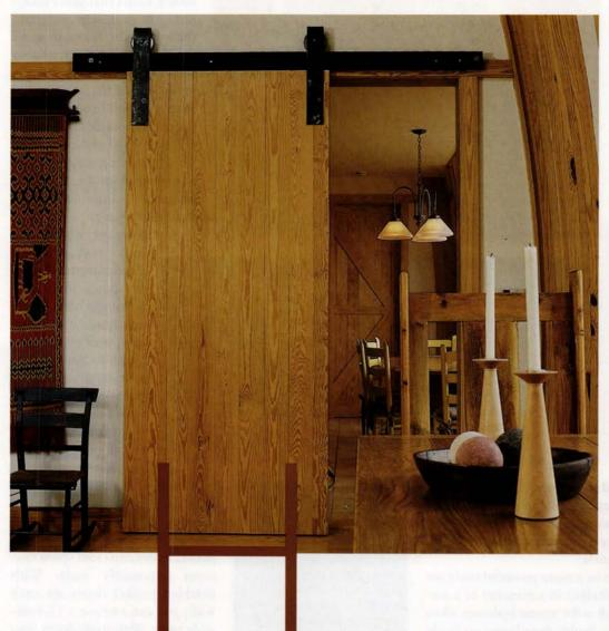
Doors built on-site, with the same materials used in other parts of the house, give a sense of continuity to a space. LEFT: A sliding barn door made with yellow pine that matches the flooring complements the rustic feel of the passageway connecting a living room with a dining room. BOTTOM: Scraps of siding from a pool house were used to build a plank door between the pool bouse and a garden shed.
