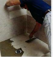
He uses a rubber trowel to smooth a layer of sandstone-colored grout over the floor tiles, letting the grout set for 10 minutes before he cleans the surface with a damp sponge.
