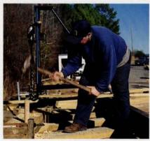
A custom-made three-legged drill press allows Graton to bore straight 2-inch-diameter holes through the overlapping lattice-truss timbers. Into these holes, crew member John Panigutti, below, pounds pegs, or trunnels, made of tough white oak. Although the trunnels were turned on a job-site lathe, Graton had their heads chiseled to resemble the drawknifed originals.
