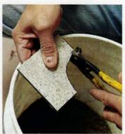
He nips a curved cut so the tile will fit snugly around the drain. Small, 4-inch-square tiles engage the pitch
