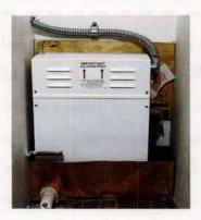
Ah—muscle-soothing, sinus-clearing, invigorating steam. Complete units for a home shower, including a generator (hidden in a closet as far as 25 feet away) and controls, cost from \$900 to \$3,700. Generators range in power from 4 to 30 kilowatts and can fill a shower with steam in less than 15 minutes. "To determine size, we take the cubic footage of the shower and factor in what it is made of—
