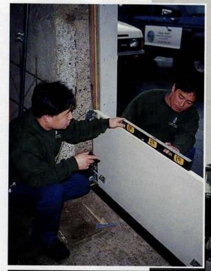
Workers from Garage Master stack the garage door panels, making sure they're level, then hinge them together along the vertical tracks in the frame.
