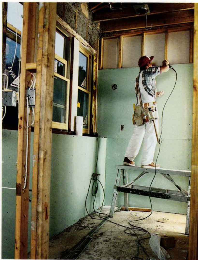
ABOVE: Ruben Moreno screws green-board (a water-resistant type of dry-wall) to the bathroom studs. BELOW LEFT: Piloting a water-cooled track saw mounted with an 8¼-inch diamond-impregnated blade, two workers slice a ¾-inch marble slab to length. BELOW RIGHT: In the bathroom, they urge a 300-pound section of marble wainscoting into position.
