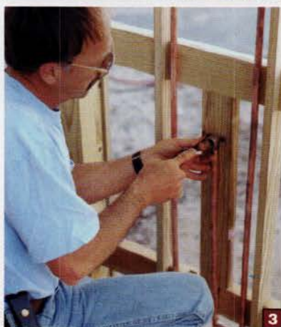
1. The frames for the shower's 5-foot-3-inch-tall double gates are mounted with a 4-inch clearance above the deck, leaving room for pickets to extend to within 2 inches of the deck. The gates swing out. 2. On the west-facing side of the enclosure, Smits lines up pickets, under a leveling stick as guide, at a height of 5-foot 9-inches. 3. Carl DeLong installs a foot-wash spigot, perfect for ensuring sand-caked toes get a thorough rinse.
