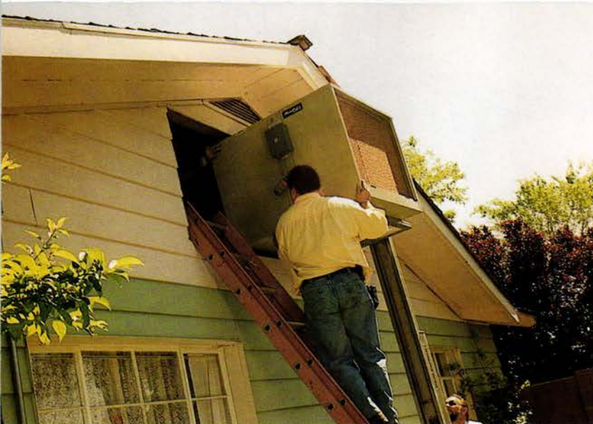
ABOVE: Evaporative coolers often score low on looks—most sit on rooftops, hang on outside walls or sit on the ground. To prevent that blight, the crew stuffs the 32-by-42-by-43-inch unit into the attic. LEFT: Moving the cooler's 6500-cfm output without slowing it down requires a big, 18-inch-diameter duct, which connects to the house's existing air-conditioning ducts.
