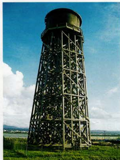
The 100-foot tower of redwood near Eureka once held aloft 331 tons of water for a lumber mill. When salvagers dismantled the structure in 1997, most of its 160 12x12 beams were recycled into a 7,000 square-foot house in La Jolla, California.
