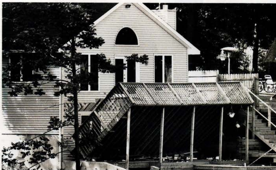
When the deck on this house near Kalamazoo, Michigan, fell during a party in 1992—killing a 57-year-old woman standing beneath it—building officials were perplexed: It appeared to have been bolted into place. A closer look revealed that the lag bolts—giant screws—had penetrated only the sheathing of the house and were not anchored into anything solid.
