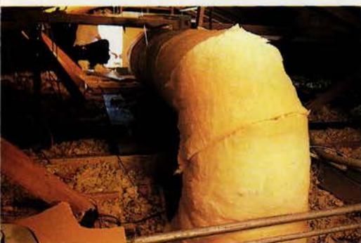
ABOVE: Evaporative coolers often score low on looks—most sit on rooftops, hang on outside walls or sit on the ground. To prevent that blight, the crew stuffs the 32-by-42-by-43-inch unit into the attic. LEFT: Moving the cooler's 6500-cfm output without slowing it down requires a big, 18-inch-diameter duct, which connects to the house's existing air-conditioning ducts.
