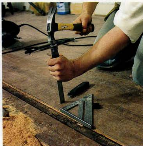
On those boards that have to be shortened, Jason Dupee scores the wood with a utility knife guided by a rafter-angle square. A few chisel blows on the score make a clean, straight cut.
