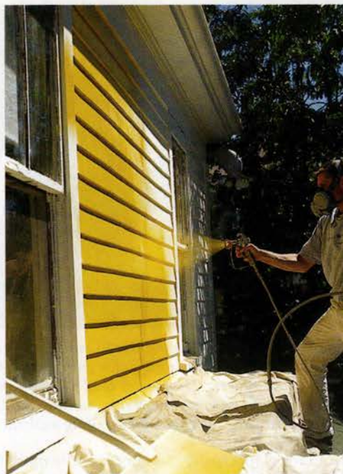
For clapboards, D'Amato chooses an airless sprayer, which pumps paint fast (but also wastes much in overspray). For detail work such as lattice, he switches to a high-volume low-pressure sprayer. It ejects less paint but is more accurate.
