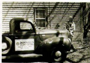
Donnell used rift-sawn scrap-pine clapboards on one of his shop buildings.
