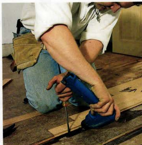
To prevent splitting, Dupee drills the tongues at an angle as he uses a screwdriver to lever a strip tight to its neighbor. He then toenails the piece every 6 inches with spiral-shanked 8d nails.
