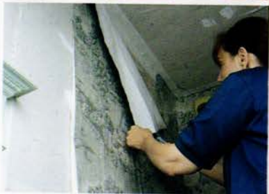
Glenna Bowman replaces wallpaper destroyed by fire at legendary House Speaker Sam Rayburn's house, now a Texas Historical Commission museum. Bowman tacks muslin to the cypress walls, top, then returns two days later to trim wallpaper for the staircase, below.
