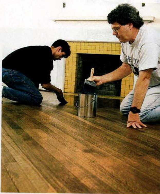
Dupee, right, and Fortin spread the first coat of polyurethane over the stained floor. They use only 4-inch China-bristle brushes because the oil-based finish would roll off synthetic filaments and leave glops. The two men always work with the grain as they brush, smoothing out bubbles and streaks in the finish with long pendulum strokes that touch just the tips of the bristles to the floor.
