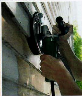
Tom Thevenin, wielding a garden sprayer, douses the house's north side with trisodium phosphate, bleach and water to vanquish dirt and kill mold and mildew. D'Amato scrubs in the solution with a stiff-bristled long-handled brush. ABOVE: The Paint Shaver at work.
