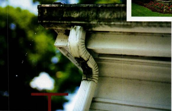
Smudged from overflowing dirty water, one of several decades-old galvanized-steel gutters at Farmstead, above, has rusted through at an elbow joint, left. Says Yates, "Every year, we spring a leak somewhere and discover a section of gutter that's buckled, bent and in rough shape."
