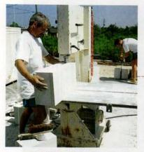
Builder Mike Havinkin runs an AAC block through a band saw, a woodworking tool. This particular block will be used in a leveling course, the first row of AAC on top of a foundation. But first, Havinkin cuts a notch to allow for a threadedsteel reinforcing rod.
