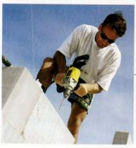
Harrison drills a hole in an AAC block to make a passage for the threaded rod that connects the rows, top to bottom—eventually tying slab to roof. Although AAC can be worked with hand tools, Poate's crew prefers power tools for ease and precision.
