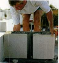
Havinkin lays the leveling course of AAC on the concrete slab foundation. He aligns the block carefully against a horizontal string that is set around the entire foundation. For this course only, traditional mortar is used to bond the AAC to the slab.
