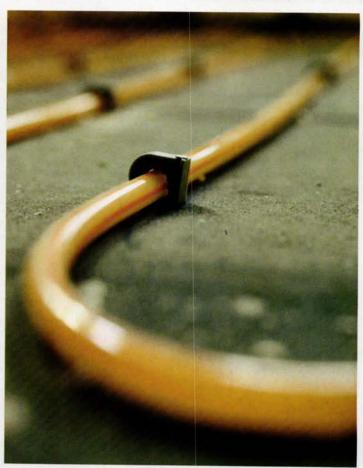
Installed correctly, radiant floor heat can give a lifetime of trouble-free comfort. Richard pressurizes the system with air or water during construction. "If somebody hits a nail through a tube, you know it right away—rather than finding out after everything's embedded in concrete."
