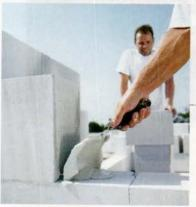
After the leveling course is set, rows of AAC stack up like toy blocks. A joint of specially formulated thin-set mortar bonds the blocks; it must measure precisely ½ inch thick to keep each row level. Masons use a trowel designed to spread exactly the right amount of the mortar.
