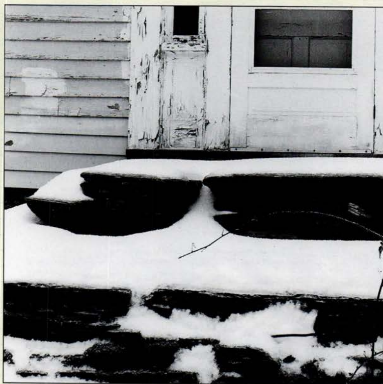
The south side of the house has taken the worst beating over the years. In addition to frayed paint and decayed clapboards, stone steps for an entryway have come loose from their moorings. The steps rest on a stone base that has become uneven. "One of the things that worries me most about this house is the marriage of stone and wood," says Klinkenborg.
