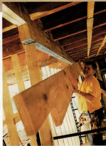
With the second LVL nailed and glued to the first, Tom hoists the final one into place. A 2x4 stud temporarily holds the planks in position during the installation.
