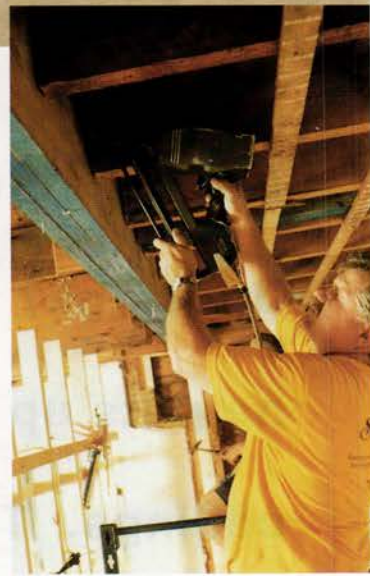
Tom nails the LVLs to each other with 3 1/4-inch nails. He fires a line of five nails from the top to the bottom of the beam section every 16 inches along the 14-foot length.
