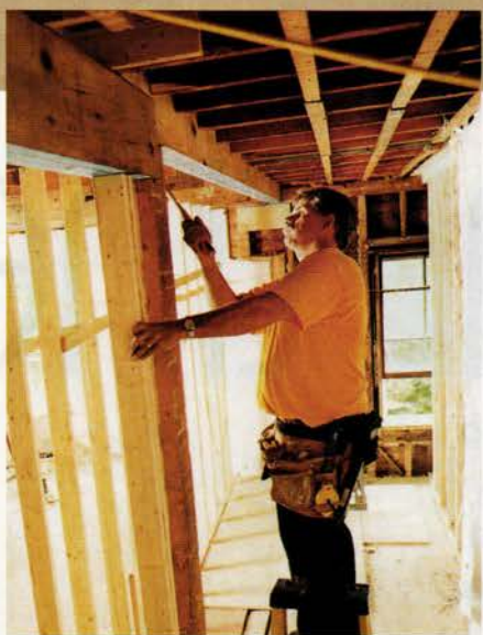
Using 3 1/4-inch nails, Tom toenails the beam to the old post. He salvaged the 4x8 timber from the wall between the original 1890 house and its 1910 addition.
