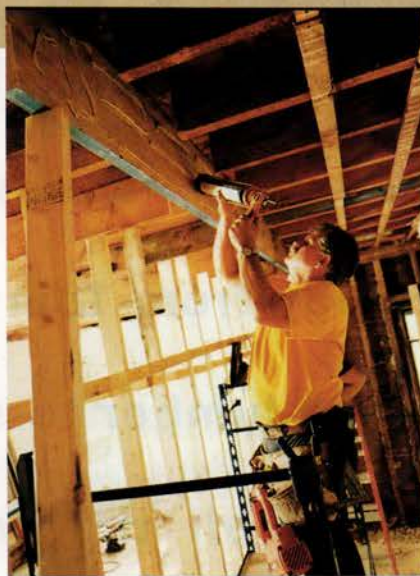
To mate the first LVL plank much more securely to the next one than nails alone would, Tom applies construction adhesive to the 11 1/2-inch-wide surface.
