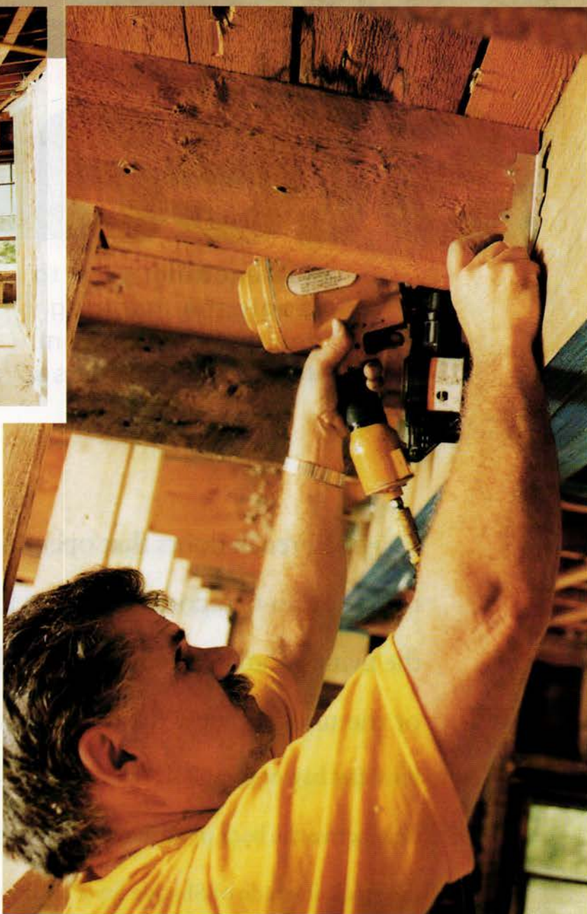
Finally, with post and beam in position, Tom goes back to the flush-framed section of the beam and installs metal joist-hangers to make a stronger connection between the 90-year-old joists and the brand-new beam.
