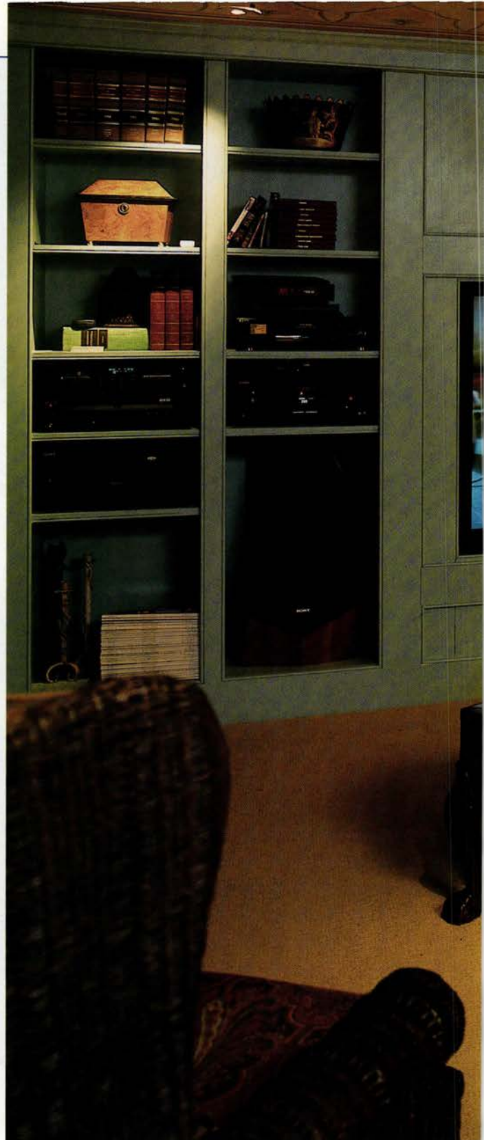
The TV cabinet's bottom panels are removable, allowing access to the TV—which rolls out on wheels—and all wires. Norm Abram and Tom Silva built the cabinet from medium-density fiberboard.
