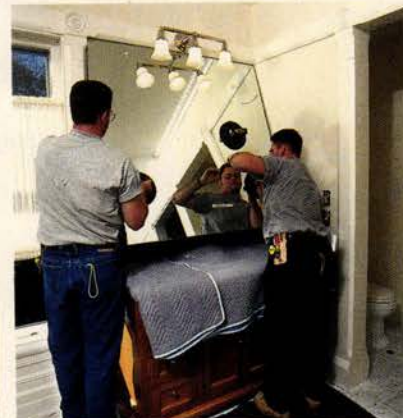
To install the frameless shower door, left, Jamie O'Brien bores a hole for a hinge screw. Made of 3/8-inch clear tempered glass, the door is held in place by two wall-to-glass hinges. The 1/4-inch-thick clear mirror above the vanity, right, is muscled into place by O'Brien, with an assist from Mike Granata, and affixed to the wall with three types of mirror mastic, adhesives formulated so they do not attack the mirror's silver coating.
