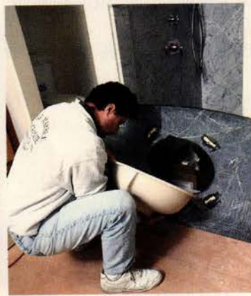
To prepare one of the cherry vanities for an undermounted sink, Julio Belloso, left, takes a "very, very careful" pass with a jigsaw to trim the frame inside so that the sink will fit. Coworker Jorge A. Cisnero, right, affixes the sink to the green marble countertop with bolts, then applies silicone caulk to the perimeter of the entire countertop underside. When the silicone sets, the whole unit will be caulked and bolted into place.
