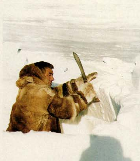
LEFT: Jack lifts a wedge-shaped snow block he has cut from the surface of the frozen inlet, creating a hole that will later become the entrance to the igloo. CENTER: After sawing a rectangular block from the snow, he prepares to position it. RIGHT: Jack uses a snow knife, also called a pana , to trim edges so the blocks lock tightly together.
