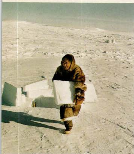
LEFT: Jack lifts a wedge-shaped snow block he has cut from the surface of the frozen inlet, creating a hole that will later become the entrance to the igloo. CENTER: After sawing a rectangular block from the snow, he prepares to position it. RIGHT: Jack uses a snow knife, also called a pana , to trim edges so the blocks lock tightly together.
