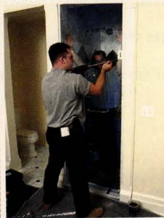
To install the frameless shower door, left, Jamie O'Brien bores a hole for a hinge screw. Made of 3/8-inch clear tempered glass, the door is held in place by two wall-to-glass hinges. The 1/4-inch-thick clear mirror above the vanity, right, is muscled into place by O'Brien, with an assist from Mike Granata, and affixed to the wall with three types of mirror mastic, adhesives formulated so they do not attack the mirror's silver coating.
