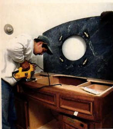
To prepare one of the cherry vanities for an undermounted sink, Julio Belloso, left, takes a "very, very careful" pass with a jigsaw to trim the frame inside so that the sink will fit. Coworker Jorge A. Cisnero, right, affixes the sink to the green marble countertop with bolts, then applies silicone caulk to the perimeter of the entire countertop underside. When the silicone sets, the whole unit will be caulked and bolted into place.
