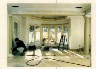
rate from the main walk," says Kaufman. In the new kitchen-family room combination (top photo), Kaufman bumped out the back wall by 12 feet and added a laminated beam supported by steel columns for strength.
