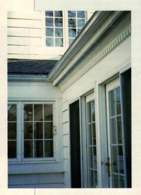
plywood sheathing at the edge of the roof, carpenters nailed 3-foot-long 2x6s to the exposed ends of the rafters, then sheathed and roofed the extension, attached a fascia board, built a soffit, put strips of decorative molding under it and attached a new gutter. "It's really simple," says Schettino. "But the look is polished, more elegant."
