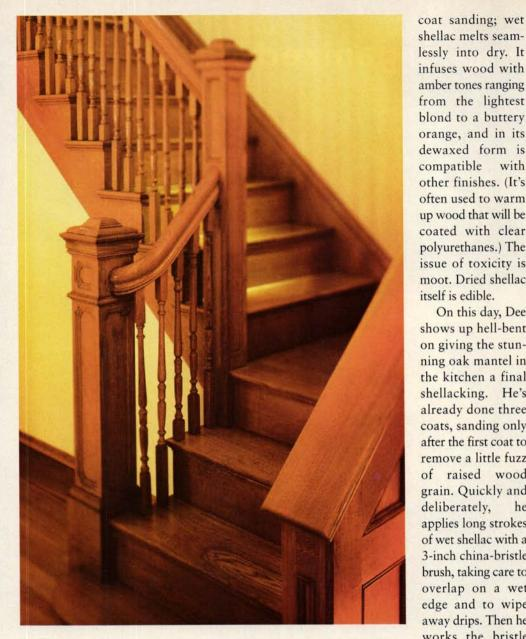
Durability determined the mix of clear finishes on the oak staircase at the Watertown house. The scuff-prone treads have three coats of oil-based polyurethane, one of the toughest finishes around. All the remaining woodspindles, hand rails, risers and newel post-is swathed in shellac, a more delicate but easily repaired coating.
