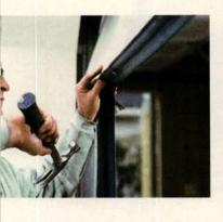
TOP: Removing a door roller requires bending out a track edge and doing a little prying. Then the axle just slips out of the hinge, MIDDLE: Raising the door relaxes the extension springs and makes them easy to take out and replace. BOTTOM: A length of soft rubber weatherstripping keeps a wood door away from the rot-inducing moisture always present in concrete.
