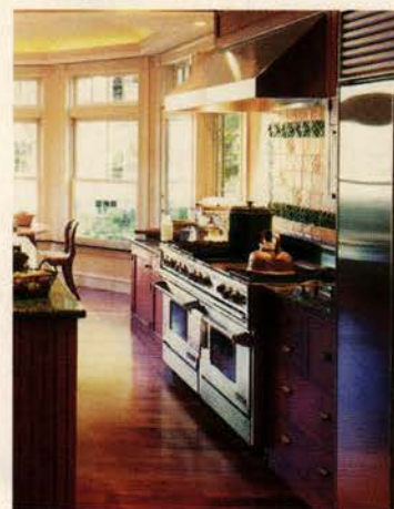
The 60-inch hood in this Lexington, Massachusetts, kitchen, below right, has an outside-mounted blower, which minimizes noise. Above left, Richard Silva holds the canopy while Charlie Silva fastens it. Above right, Charlie mounts the blower housing over the 10-inch exhaust opening.
