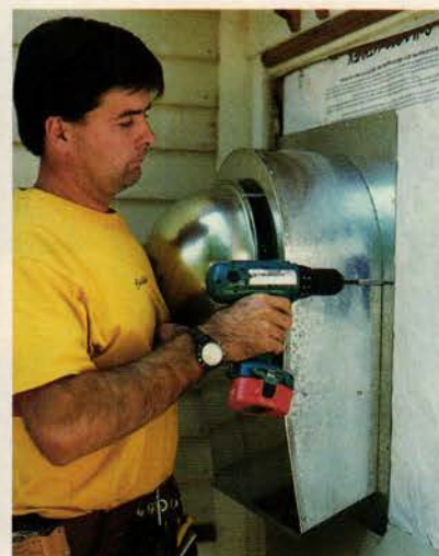
The 60-inch hood in this Lexington, Massachusetts, kitchen, below right, has an outside-mounted blower, which minimizes noise. Above left, Richard Silva holds the canopy while Charlie Silva fastens it. Above right, Charlie mounts the blower housing over the 10-inch exhaust opening.
