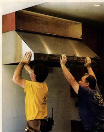
The 60-inch hood in this Lexington, Massachusetts, kitchen, below right, has an outside-mounted blower, which minimizes noise. Above left, Richard Silva holds the canopy while Charlie Silva fastens it. Above right, Charlie mounts the blower housing over the 10-inch exhaust opening.
