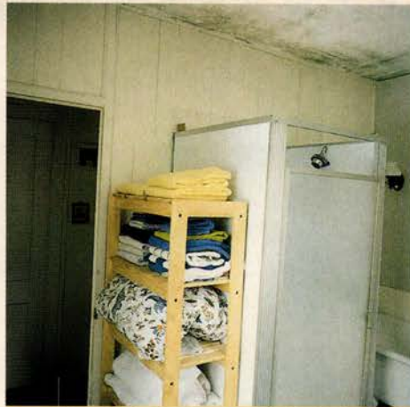
LEFT: Despite the bathroom's 9½-foot ceilings and abundant natural light, an old shower stall and poor ventilation have led to excessive mildew. RIGHT: The cramped tub and toilet arrangement throws off the room's proportion.
