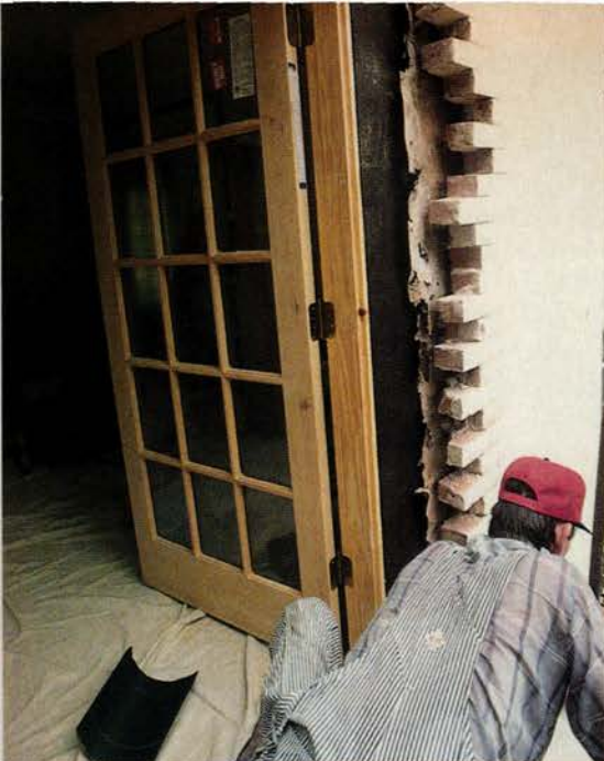
Black strips of building felt stop water from getting between the sheathing and the framing.
