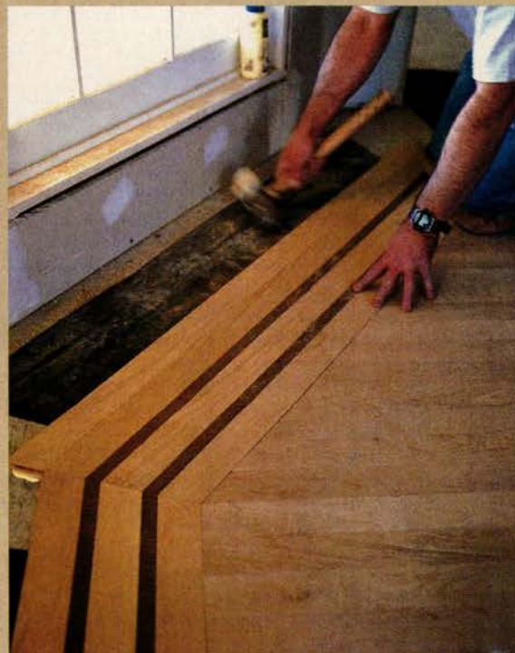
TOP LEFT: The thump of a rubber-faced mallet echoes through the house as Geider Silva whacks the floor nailer while his father arranges the white-oak strips. LEFT: Carlos cuts the corners to make the octagon that mirrors the room's shape. ABOVE: After much trial and error to find the right angle, Carlos taps in a perfectly fitted border strip.
