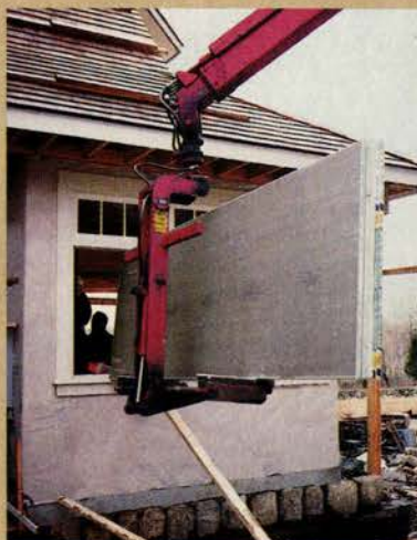
ABOVE: A mechanical arm moves the 96-pound sheets through any available opening. RIGHT: Installing the sheets, however, requires sheer muscle power as, from right to left, Vince McVay and Peter Garre hold while Tim Grady fastens.
