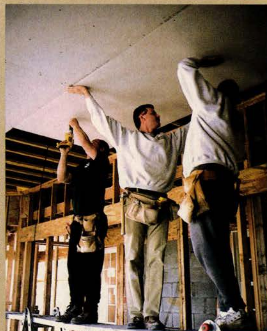
ABOVE: A mechanical arm moves the 96-pound sheets through any available opening. RIGHT: Installing the sheets, however, requires sheer muscle power as, from right to left, Vince McVay and Peter Garre hold while Tim Grady fastens.
