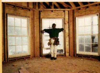
ABOVE: Fortunately for carpenter Phil Whipple, heavy sash can be removed to ease the window frame installation. BELOW: After fastening the frames, Whipple replaces the sash in just seconds.
