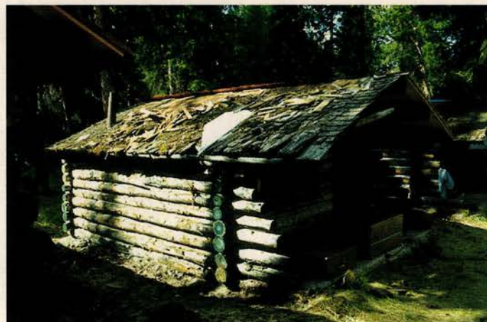
The rustic 80-year-old guest cabins suffer from rotting roofs and logs.
