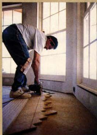
TOP LEFT: The thump of a rubber-faced mallet echoes through the house as Geider Silva whacks the floor nailer while his father arranges the white-oak strips. LEFT: Carlos cuts the corners to make the octagon that mirrors the room's shape. ABOVE: After much trial and error to find the right angle, Carlos taps in a perfectly fitted border strip.
