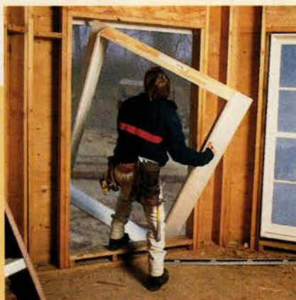
ABOVE: Fortunately for carpenter Phil Whipple, heavy sash can be removed to ease the window frame installation. BELOW: After fastening the frames, Whipple replaces the sash in just seconds.
