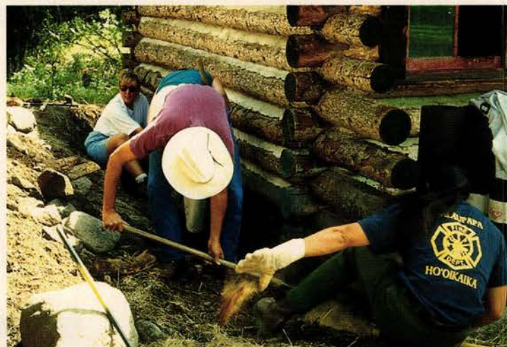
To put the cabin back on a firm footing, volunteers dig out a punky log.
