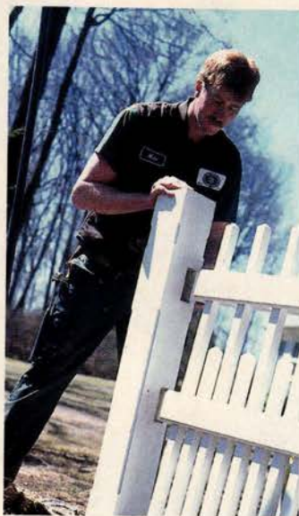
To extract a damaged post from its hole, Mike Sludock pulls and pushes the cedar 6x6 to loosen the soil.
