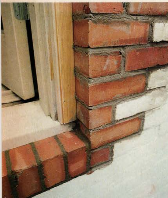
Once the door is in, new bricks are rewoven over the exposed sheathing and sill.
