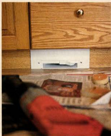
Crumbs swept into the mouth of a power dustpan (which is mounted flush with the floor) disappear at the touch of a button.
