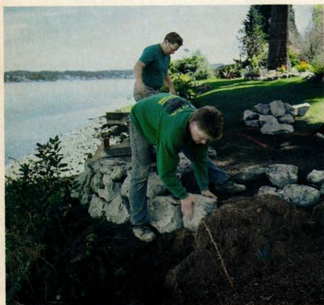
Zwieg builds a retaining wall for the beach stairs, following the route on the lawn that Robin Rodgers, rear, mapped out earlier with orange spray paint.
