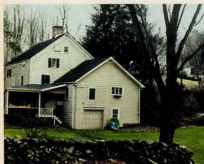
LEFT: Before renovation, the house sported an ill-conceived 1950s kitchen addition with a rarely used garage and a rickety porch. RIGHT: The first stage was to remove the addition without endangering the 18th-century post-and-beam construction.
