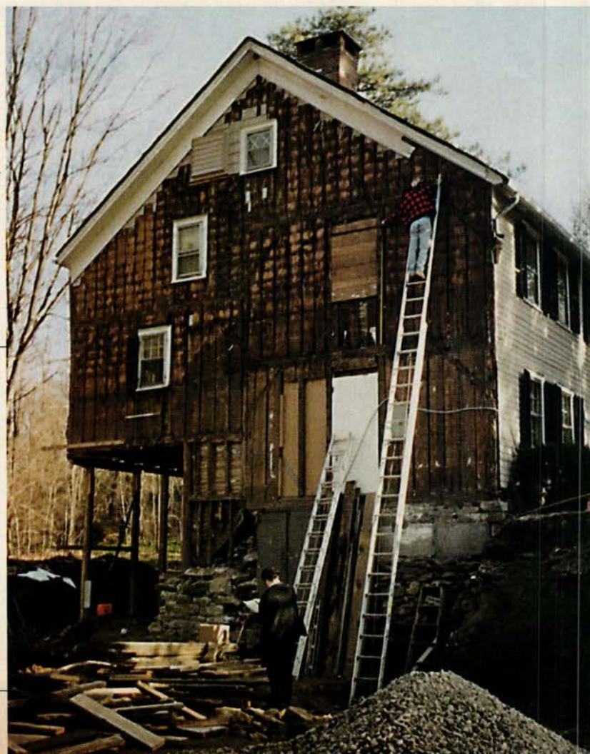
LEFT: Before renovation, the house sported an ill-conceived 1950s kitchen addition with a rarely used garage and a rickety porch. RIGHT: The first stage was to remove the addition without endangering the 18th-century post-and-beam construction.
