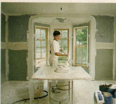
ABOVE: With the ceiling, corners and seams already covered, Bob DeFranzo mixes a fresh batch of plaster for the Silvas' dining-room walls. BELOW: As he loads his hawk, he knows he has about 45 minutes before this batch will harden.
