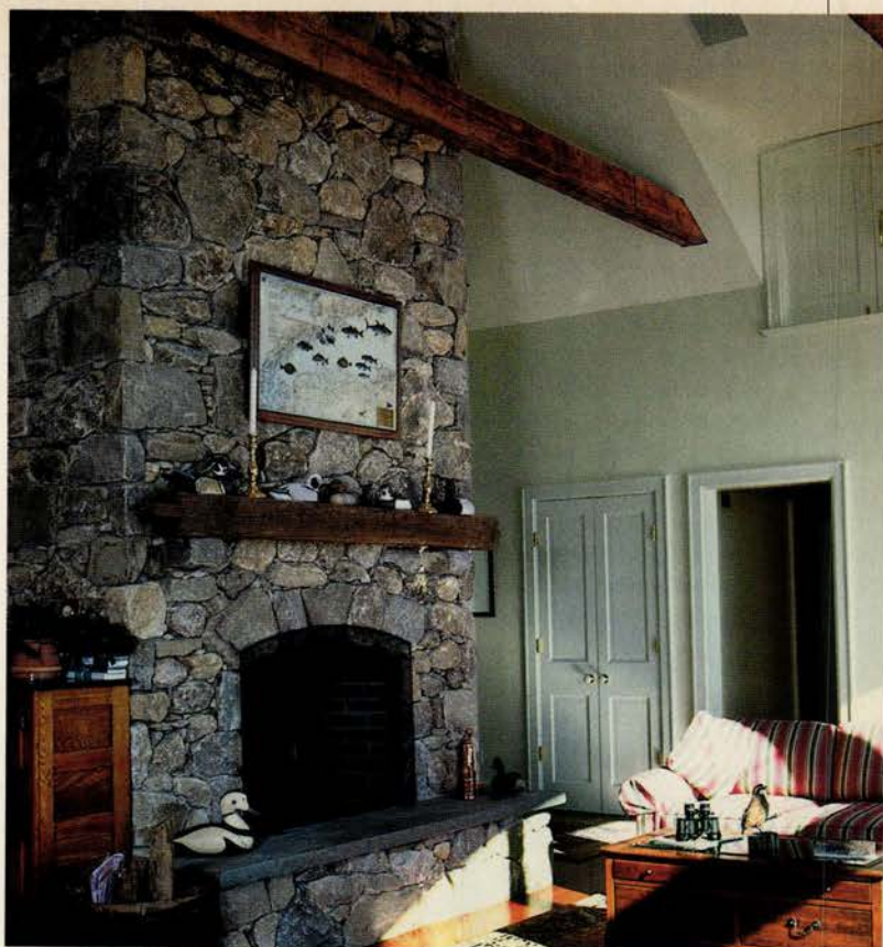
Built with 100 tons of fieldstone and concrete block, the exposed chimney sports a plain wood mantel shelf reminiscent of the ceiling beams.
