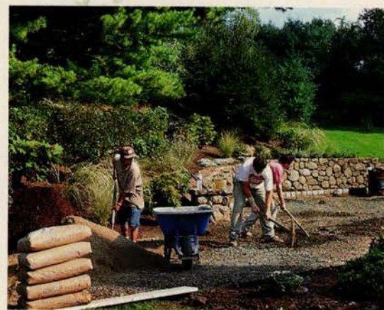
TOP: "The plantings are casual and lovely," says landscape architect John Geiger of his overall scheme for an English-style garden. ABOVE: Workers dig a trench at the perimeter of the graveled turnaround, in which they will lay a cobblestone border.
