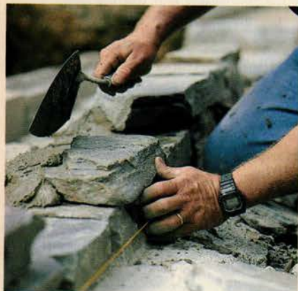
ABOVE: With each new course of stone, landscaper Roger Cook makes sure to cover the joints of the course below and to keep the mortar away from the wall's face.
