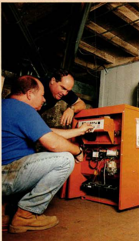
T.O.H. plumbing and heating consultant Richard Trethewey and plumber Richard Bilo ready the boiler in the Salem house project to provide hot water and warm air and floors.
