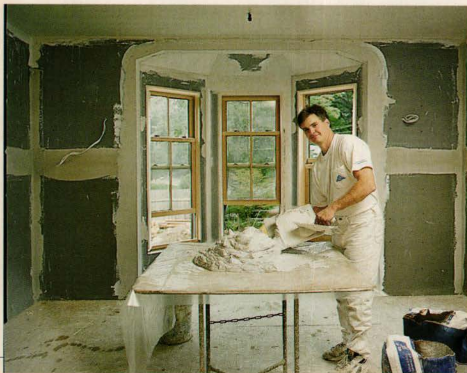
ABOVE: With the ceiling, corners and seams already covered, Bob DeFranzo mixes a fresh batch of plaster for the Silvas' dining-room walls. BELOW: As he loads his hawk, he knows he has about 45 minutes before this batch will harden.
