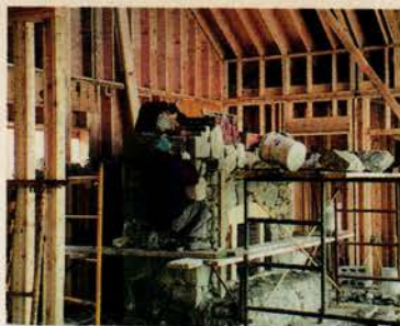
Built with 100 tons of fieldstone and concrete block, the exposed chimney sports a plain wood mantel shelf reminiscent of the ceiling beams.
