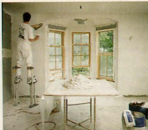
ABOVE: With sweeping arcs of his trowel, DeFranzo moves the plaster from table to hawk to wall. He finishes all the hard-to-reach spots on stilts. BELOW: A damp felt brush and a trowel perform the final smoothing: no sandpaper needed.
