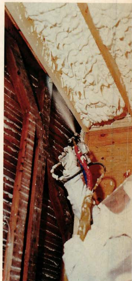
This spray-in foam insulation, known as Icynene, emits no toxic gases, reduces the need for roof vents, and can seal otherwise inaccessible air leaks in houses.
