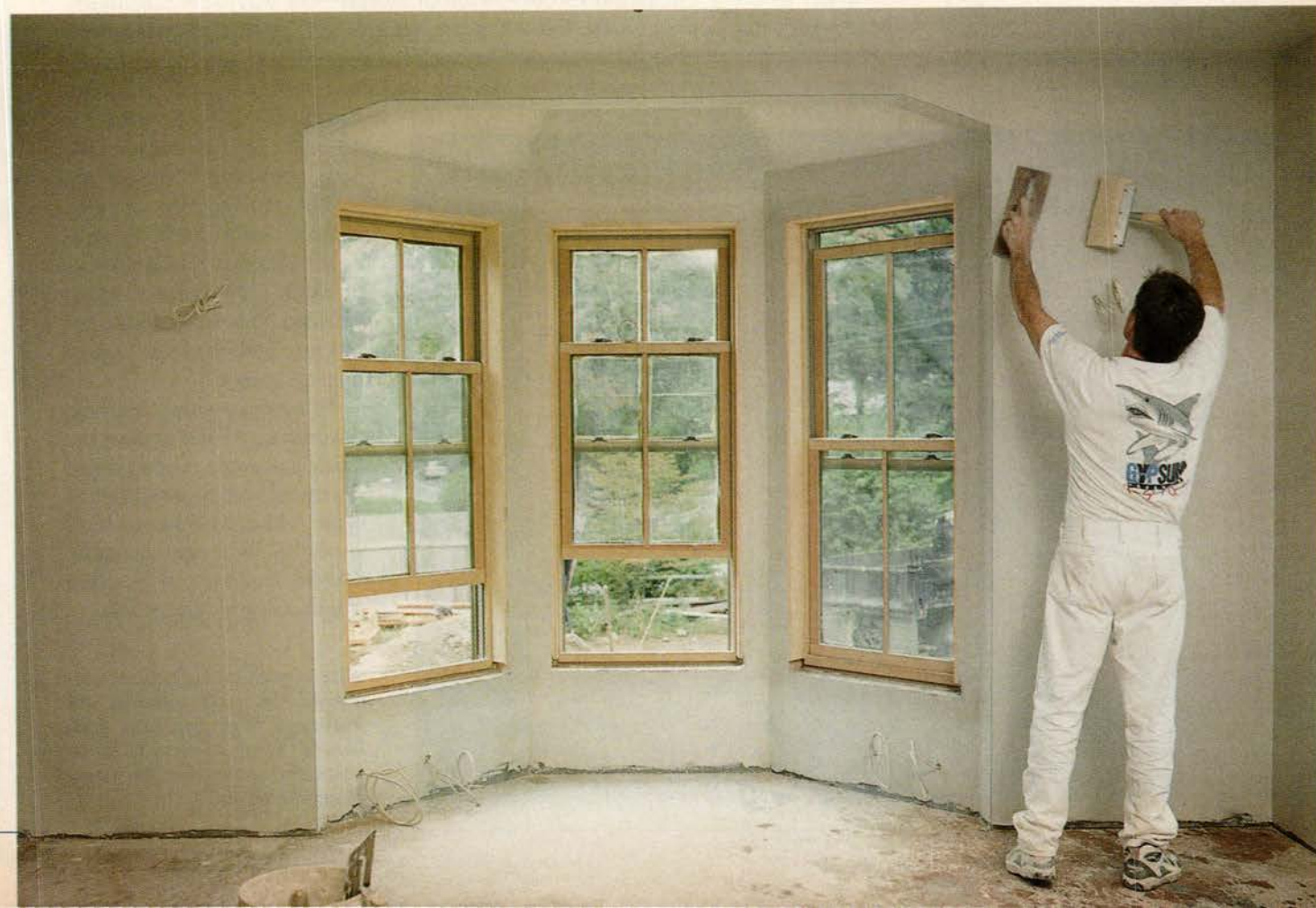
ABOVE: With sweeping arcs of his trowel, DeFranzo moves the plaster from table to hawk to wall. He finishes all the hard-to-reach spots on stilts. BELOW: A damp felt brush and a trowel perform the final smoothing: no sandpaper needed.
