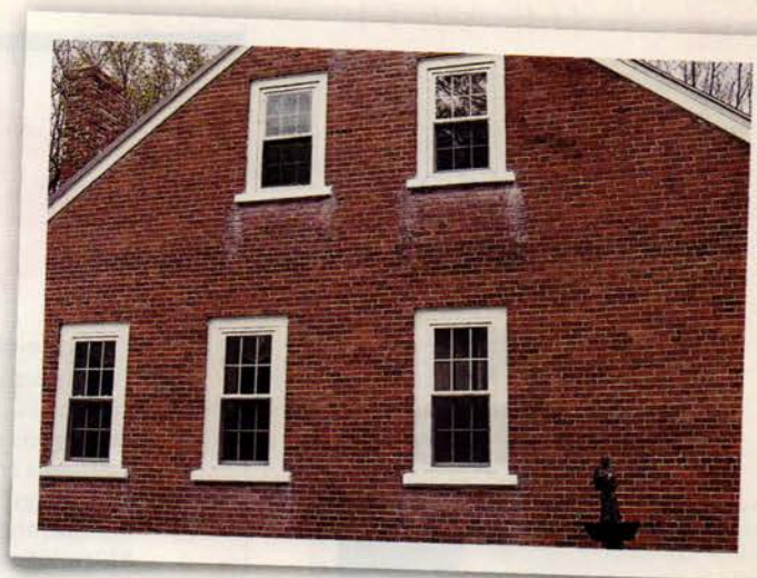
Pigment-laden runoff has stained the old porous brick below these windows. A thorough soaking and a gentle cleaning of the brick may be all that's needed to get rid of the stain.
