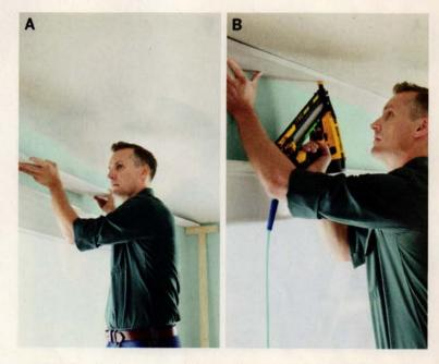
TIP The beams need to be tight to the ceiling at the joists, but any gaps that appear between joists will be covered later by the molding.
