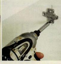
5] **Install the mounting plate.** Remove the mounting plate from the hinge. Align its three screw holes with the intersecting layout lines on the side panel. Using the self-centering bit, drill pilot holes through the plate's holes, then attach the plate with the 5%-inch #6 screws, as shown. Do the same for each hinge.
