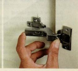
6] **Mount the door.** Hold the door in the open position and hook the hinges onto their mounting plates, as shown. Press on the bars to snap them in place against the plates. Now close the door and check the reveal. To see how to fine-tune the hinge and get perfect door alignment, go to thisoldhouse .com/novdec2013.
