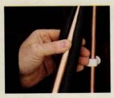
□ Insulate pipes: Add foam insulation to any exposed plumbing to keep the lines from freezing when the cold sets in.
