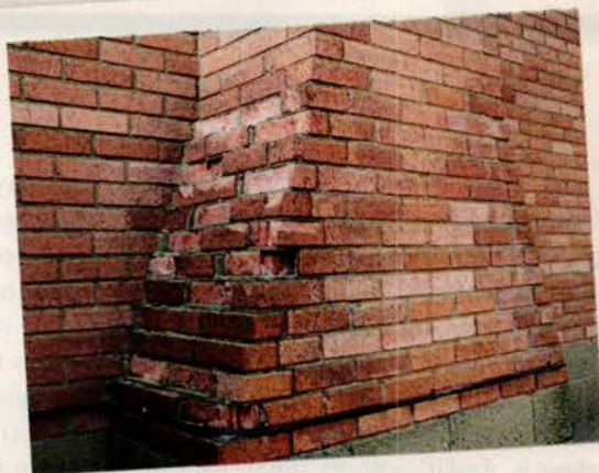
If this chimney's shoulder bricks had been sloped, water would not have soaked in and frozen, causing this spalling.
