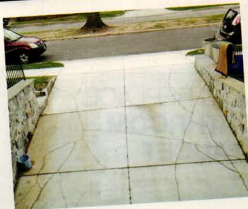
A web of unsightly cracks in a new concrete driveway indicates that something went wrong during the prep or pouring phase or with the curing shortly thereafter.
