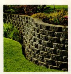
This serpentine wall, made of interlocking concrete blocks, has the look and durability of stone, without the high installation cost.
