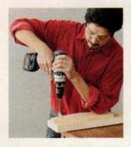
3 MAKE THE HANDLE OPENING Using a 1-inch paddle bit, drill a hole 11/2 inches down and into the middle of each side for the dowel handle.
