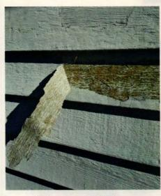
This solid-color stain peeled off in sheets, either because it was applied over a dirty, poorly prepared surface or because moisture migrated through the wood from behind the siding.
