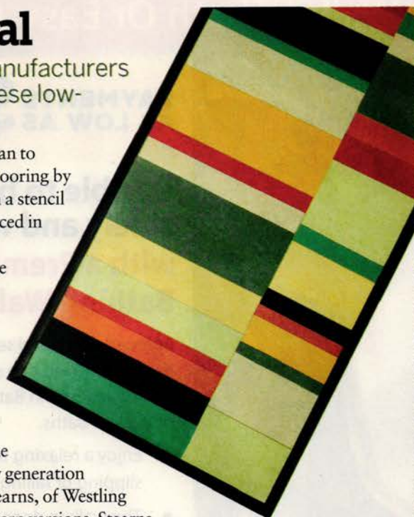
Linoleum rectangles come together to form a colorful, carefree rug. The sloped reducer edging prevents tripping.
