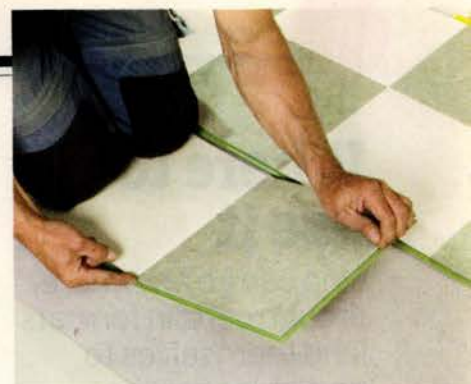
Install click-together tiles at a 15- to 20-degree angle and they'll snap right in.
