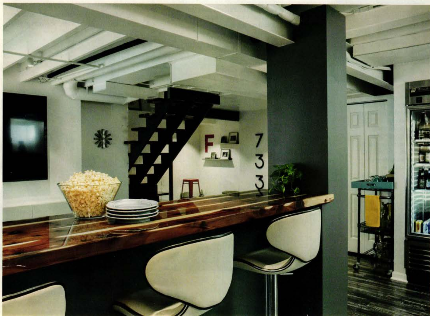
ABOVE: Bill turned the metal support column into a functional detail by boxing it in with 1×4 pine boards, making it a dividing wall that holds a TV on one side and lighting on the other. BELOW: Neutral wall colors, open-riser stairs, and a white exposed ceiling keep the walk-out basement feeling bright.
