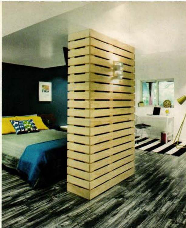
ABOVE: Bill turned the metal support column into a functional detail by boxing it in with 1×4 pine boards, making it a dividing wall that holds a TV on one side and lighting on the other. BELOW: Neutral wall colors, open-riser stairs, and a white exposed ceiling keep the walk-out basement feeling bright.
