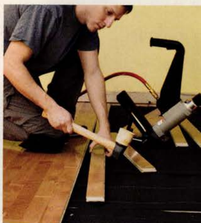
A mallet racks boards together; the pneumatic nailer secures them.
