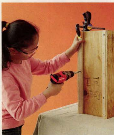
> The sides of the form , made from rough, exterior-grade sheathing, impart the grain onto the concrete as it cures.
