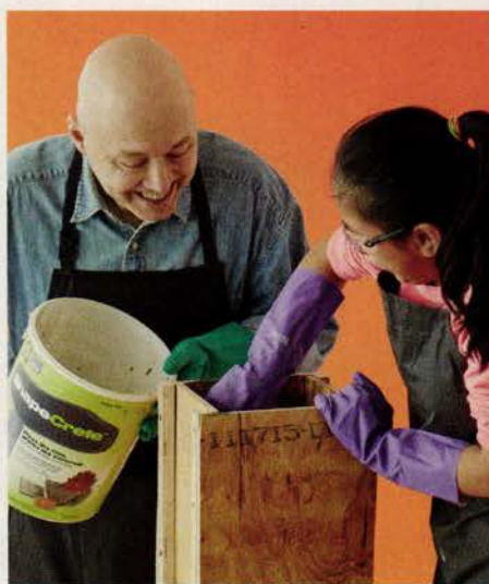
> The concrete is fiber-reinforced to minimize cracking. The team packed it onto the walls, a handful at a time, until the sides were about 1/2 inch thick.
