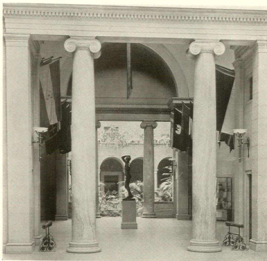
In the Rotunda, the columns are of Maryland marble; the floor and bases are of Tennessee.
