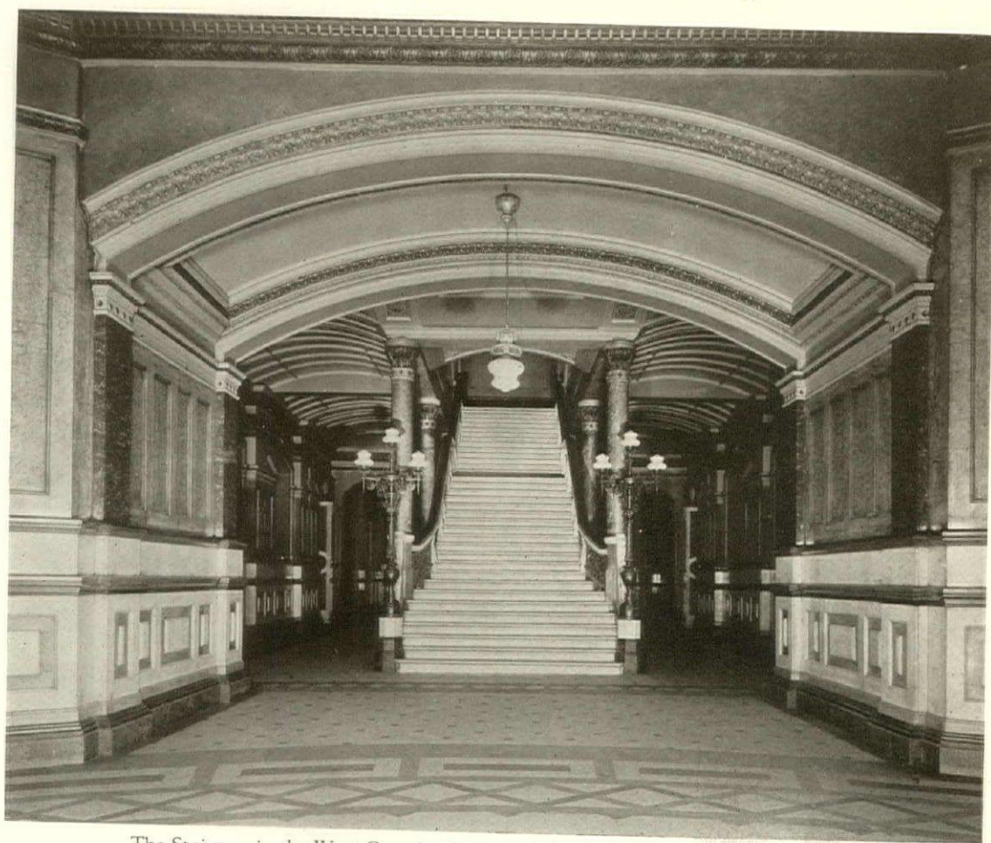
The Stairway in the West Corridor, built entirely of marble on a framework of iron. Notice the handsome columns.
