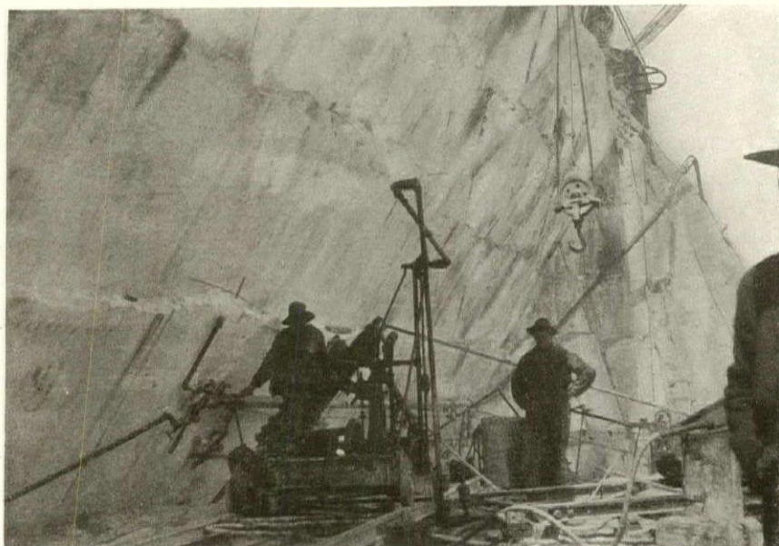
Channeling marble in one of the Colorado quarries.
