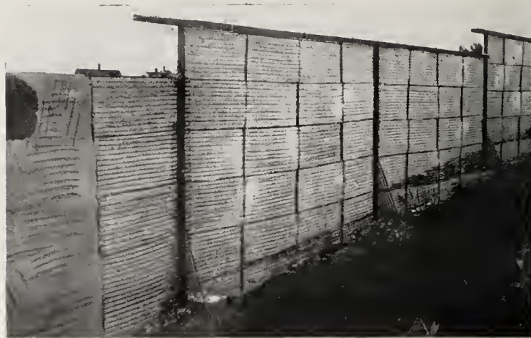
Photo of the New Fence.
